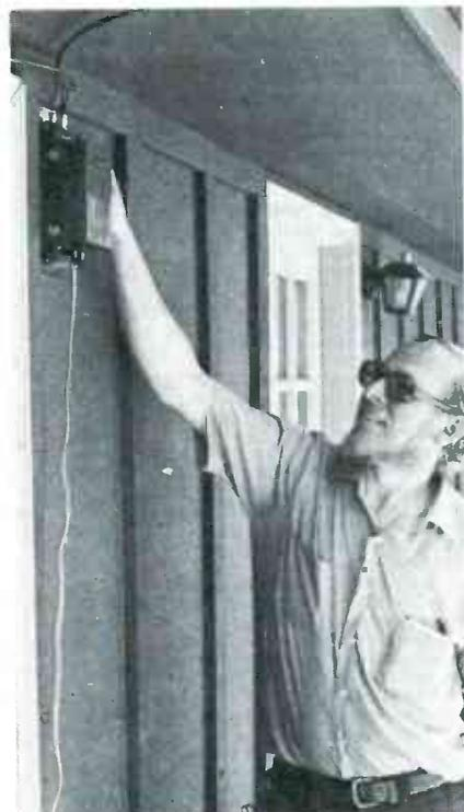
The PS-24 power supply needs to be located near a source of 120-volt power. In this installation, it was under the eaves of a house near the foot of the hill where the antenna was mounted. The unit supplies 24 volts AC to power the CLA's and the remote antenna preamplifiers.
