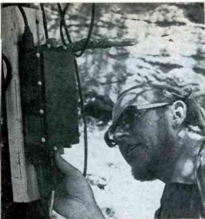
A CLA mounted on a tree provides a convenient test point to check the signal levels. Mr. Benbow is shown connecting a signal-lever meter to the -20-dB test connector.
