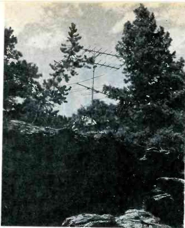
From top to bottom, the antennas are: two horizontally-stacked high-band yagis for Denver channels 7 and 9; a single low-band yagi for Denver channels 2, 4, 6, and FM; and a single high-band yagi for Colorado Springs channels 11 and 13.
