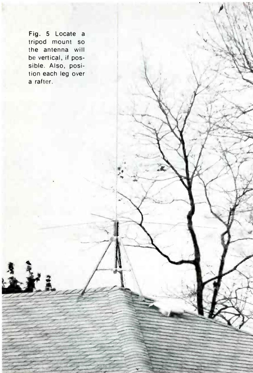
so all the lag screws bite into solid wood. This is most likely at a spot where a pair of rafters join the ridge. You can "probe" for solid wood by hammering a slim screwdriver bit or a nail-set punch into the roof till you find solid rafter. (Be sure it's not just the plywood roof sheathing.) Holes made this way and not used are easily sealed.
