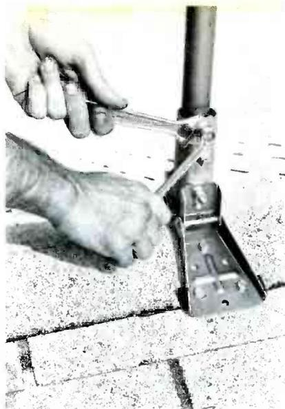
Fig. 9 Screws in the saddle mount hold the mast firmly, after the guys are all in place. Two wrenches are necessary because of the lock nut.
