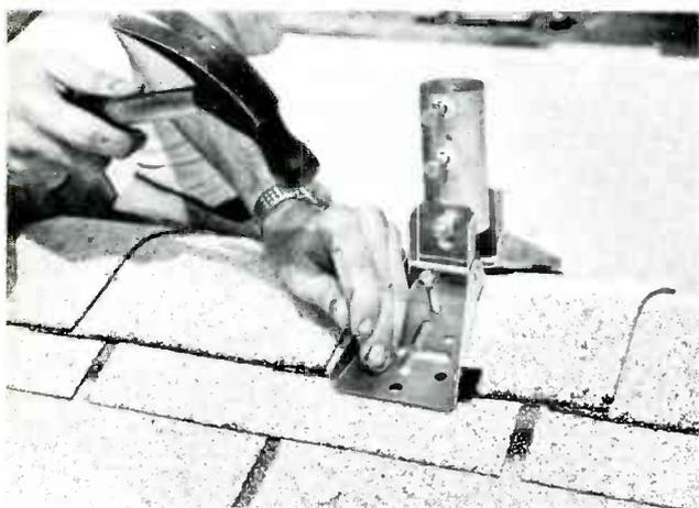
**Fig. 3** Use a center punch to dent the roofing where the screws will go. Soft wood needs only a small starter hole; but for oak or other hard woods, make a complete hole (just slightly smaller than the screw for a tight fit without splitting the wood).
