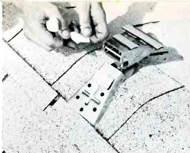
**Fig. 2** On the bottom of the saddle mount, cover the screw holes with self-sticking tape, which prevents water from entering.
