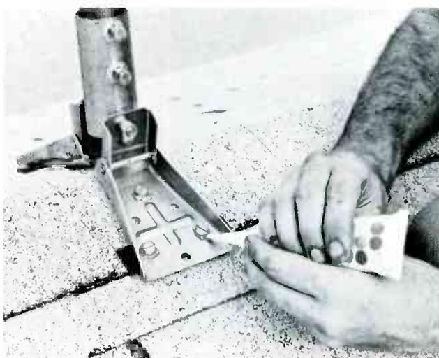
**Fig. 4** After the mount is fastened in place, apply caulking to the edges of the mount and to the screw heads. This prevents leaks.
