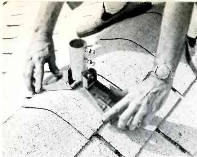
**Fig. 1** Locate a spot at the ridge where two rafters meet, so all the screws can bite into solid wood. This is a saddle mount.
