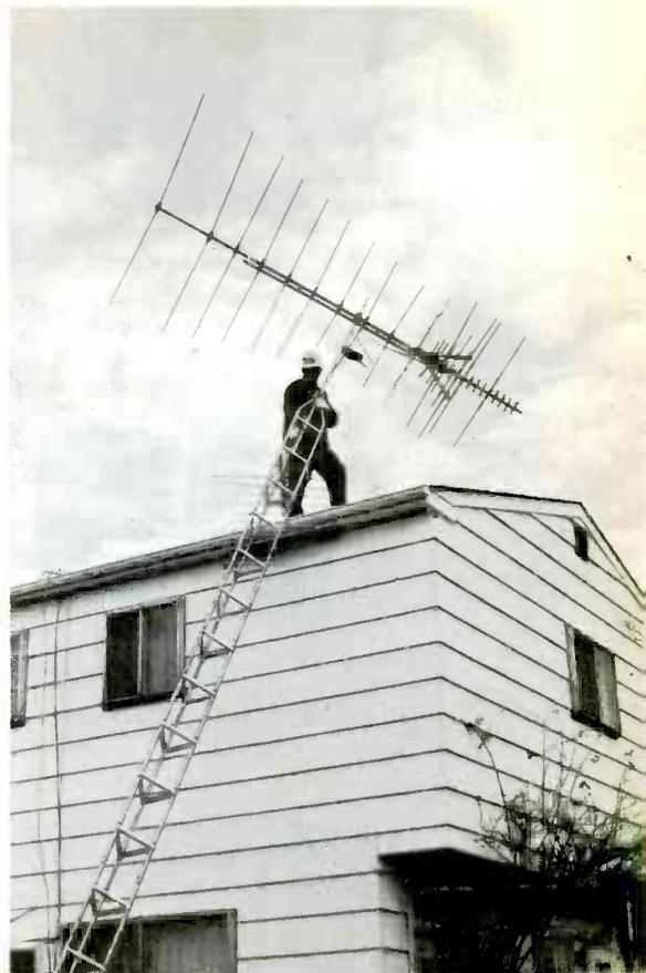
Fig. 8 The man on the roof lifted the assembled mast and antenna, connected a safety rope to prevent it from falling accidentally, and both men positioned the tower approximately where it should go.
