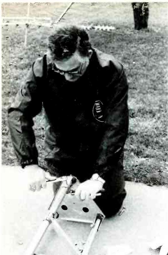
Fig. 3 The base plate is bolted securely.
