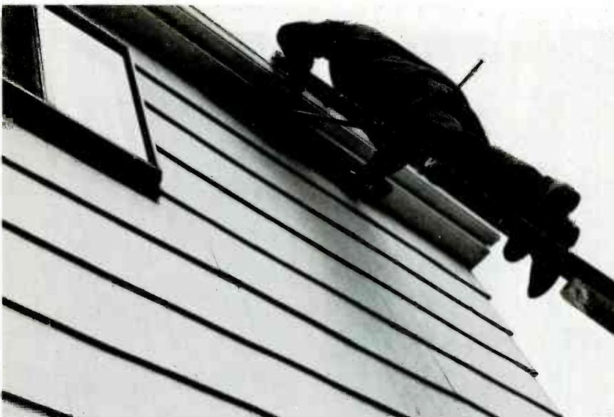
Fig. 7 Secure the 2X4 to the house, using the nails and lag screws.
