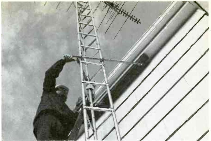
Fig. 9 A tower bracket was fastened to the tower using "U" bolts, and to the 2X4. Now, the tower was reasonably secure, but not perfectly vertical.
