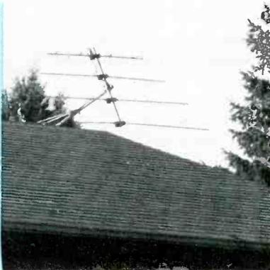
The antenna was undamaged, but the tripod mount pulled loose during a strong storm. Nails were probably used instead of lag screws to anchor the tripod feet.
