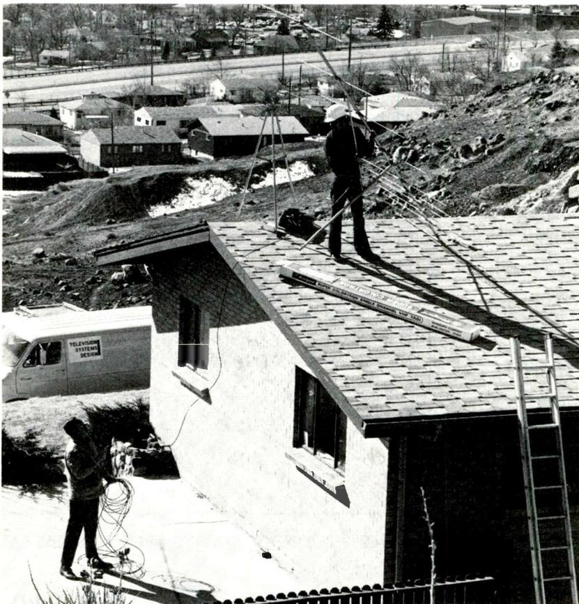
A typical home-antenna installation uses a tripod roof mount with 75  $\Omega$  coaxial cable downlead.
