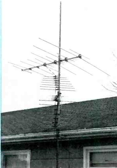
This tripod roof mount and rotor survived a windstorm safely, but the antenna suffered bent elements and a broken 300  $\Omega$  twin lead.
