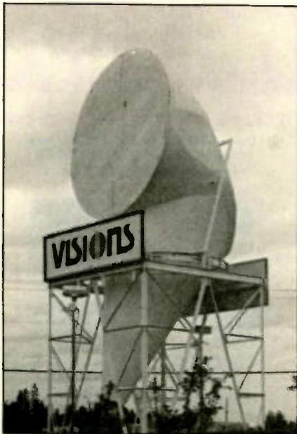
The farther north the satellite receiving site is, the lower the *look angle*. In Anchorage, Alaska, where the look angle is just above the horizon, ground clutter noise could be significant if an ordinary dish-type reflector is used. A highly directional antenna works better in this situation.
