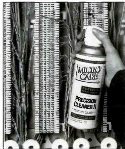
available non-CFC contact cleaner that can effectively replace the use of CFC-113. It is non-conductive, will not burn, will not attack plastics, and cannot harm operating machinery.
