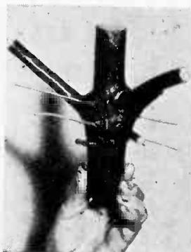
An innocent-looking arbutus tree, behind which the wires seemed to pass was, in reality, growing completely around the wires. During wet weather, the saturated wood caused the wire's resistance to change
