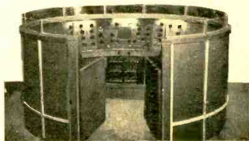
The new control console after installation.
