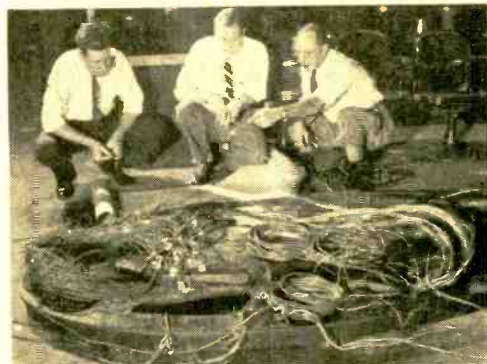
Martin Bender (right), designer, plans wiring and installation with Planetarium staff.
