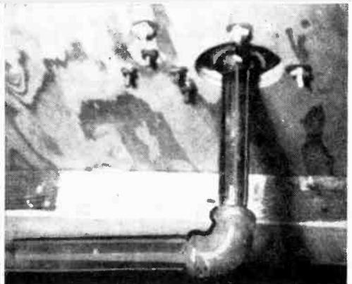
Bottom view of the motor and gear box mounting showing the crank and pipe to the garage door in the closed position. Note microswitches.
