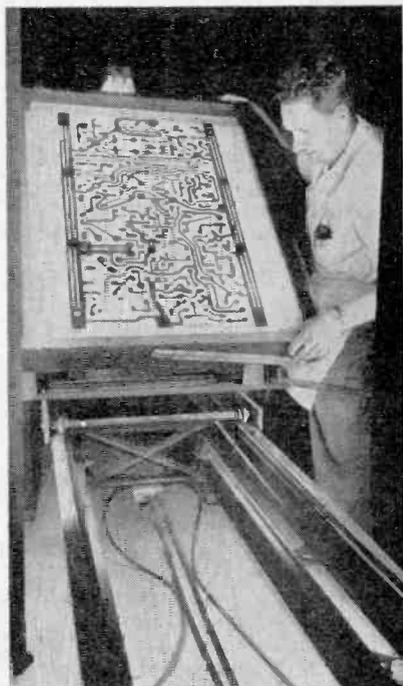
Large drawing of circuit layout is photographed with huge camera that reduces it to actual size negative. "Picture" is then printed on aluminized plastic sheet.
