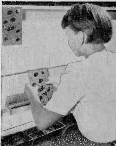
Final assembly on printed circuit layout is done by hand. Increased output has enabled firm to hire additional employees.
