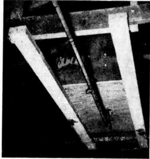
bled, mount the gear box on a piece of 5-ply plywood, 28 inches wide and 36 inches long. Cut a hole in the center of the plywood and bolt the gear box into position. Bolt a 2 x 4 along one end of the plywood, and add another piece of plywood in an upright position to the 2 x 4. This is the base for the motor.
