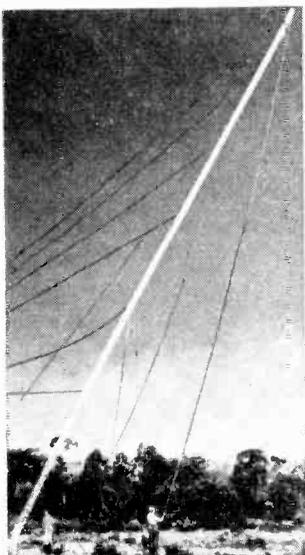
erected in the photo. Made by *Alprodeco, Inc.*, Mineral Wells, Texas, the light weight tower is assembled from six-foot sections and raised with another section of aluminum tower acting as a boom. Five men did the job in one day. Similar towers have been installed in many areas.
