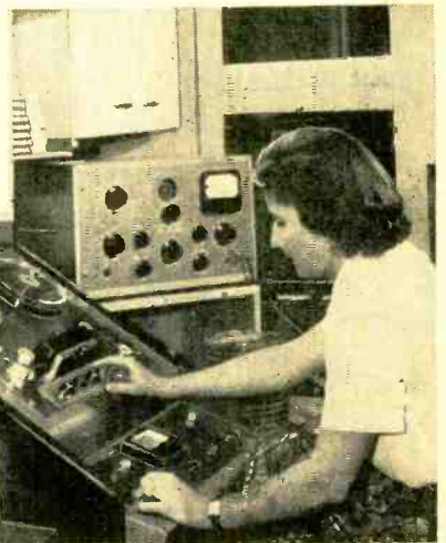
The final visual inspection of the tape is made by skilled operators who use fluorescent lighting boxes.
