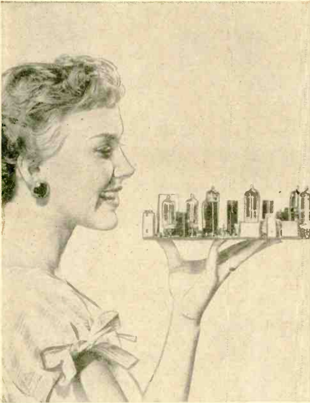
This printed circuit section represents approximately 50 per-cent of the complete chassis and is produced by automatic machines. Result is lower cost TV set.
