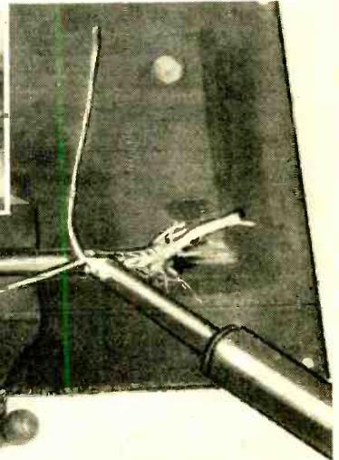
Wrap a ground wire around the braided cable and solder the wire to the shield. Be careful not to use too much heat on the center insulation as the cable will melt and short out the circuit.
