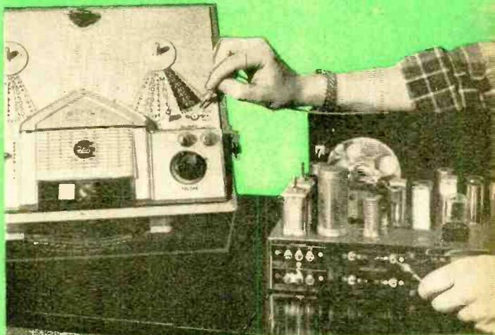
A phonograph using a high-level pickup (crystal or ceramic) may be taped by feeding its signal into the machine's high-level jack. Phonographs using low-level pickups (magnetic) should feed into a preamplifier-equalizer and then into the tape machine. A low-level magnetic phono signal may be fed into the tape recorder's low-level jack, but this does not assure proper phono equalization and is not recommended.
