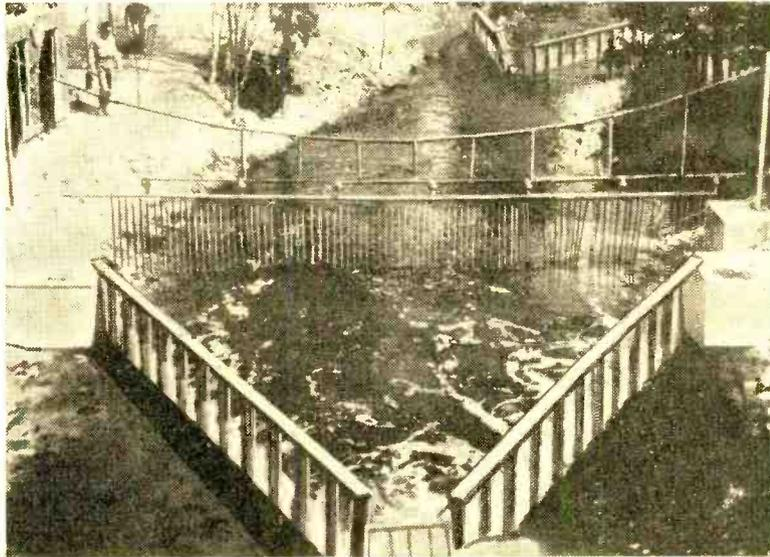
**Electrical weir** at Carp Creek, Mich. (left) is located between two mechanical weirs used in checking the effectiveness of this barrier. Lampreys, which prey on smaller fish, are killed by its charged electrodes as they attempt to pass through on their way to spawning grounds.
