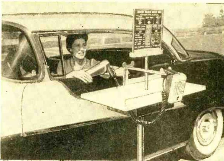
When the customer places an order for "hamburger with," this robot "car-hop" accepts the order, relays it to the kitchen, and delivers the food.
