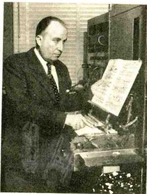
**Dr. Olson translates** musical score into punched code on "typewriter" keyboard of the Synthesizer (above). The machine converts code to sound recorded by cutter on lower disc (below). Upper disc combines tracks in simultaneous playback.
