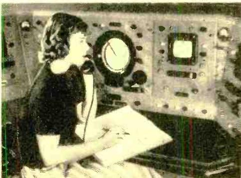
Storm tracking by radar is the latest all-electronic addition to the weatherman's arsenal. With equipment at left, the Signal Corps maps cloud movements within a 200-mile distance from transmitter.
