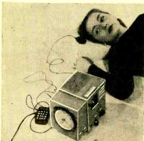
You can learn while relaxing if you have a "Memory Trainer" developed by Modernophone, Inc., 30 Rockefeller Plaza, New York 20, N. Y. A cartridge, containing a message, is inserted in the unit. It will play its contents, as controlled by a timer, through a built-in amplifier and speaker. Private earphones can be used, if preferred. Messages may also be recorded with the same device.
