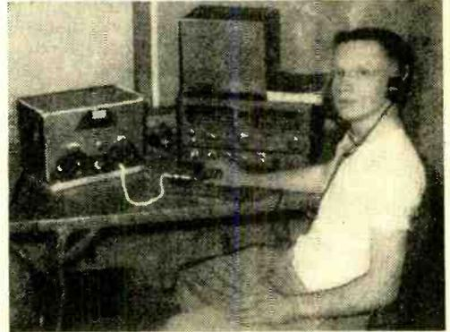
**Fred Beyer, KN9HFP**, made 200 contacts in 5 states in five months as a Novice. His transmitter is a DX-20 feeding a dipole; his receiver is an NC-98.
