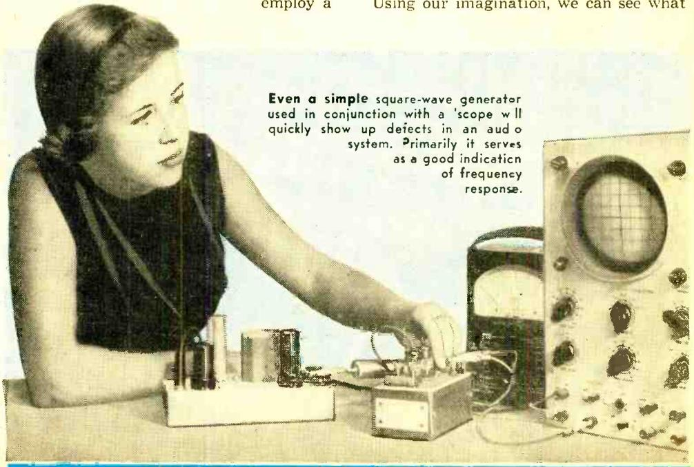
Even a simple square-wave generator used in conjunction with a 'scope will quickly show up defects in an audio system. Primarily it serves as a good indication of frequency response.
