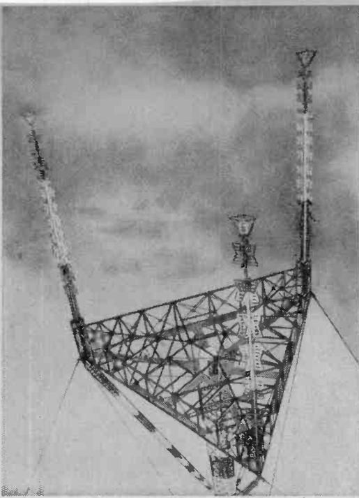
**Unique TV transmitting tower** being erected in Baltimore (left) bears a triple antenna, giving it a candelabra effect. The entire weight of the 900,000-pound structure, 729 feet tall, will be borne on legs made of U. S. Steel's new T-1 structural steel. Baltimore's three TV stations will each occupy one of the corners with a 107-foot antenna.
