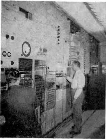
**Radio Australia's** main switchroom at Broadcast House, Melbourne, is shown above. A number of half-wave stacked arrays with reflectors mounted atop 210'-high steel towers make up the antenna system.
