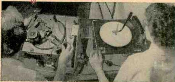
**Mechanical and operational test** involves simulation of in-use conditions. The tester checks the underside for wiring, clearances, welds and solder joints. Flipping it, she checks for freedom of all moving parts. Then she runs through intermixed 7", 10" and 12" records in several orders to check size and speed selection. "Speedminder" control is tested as well.
