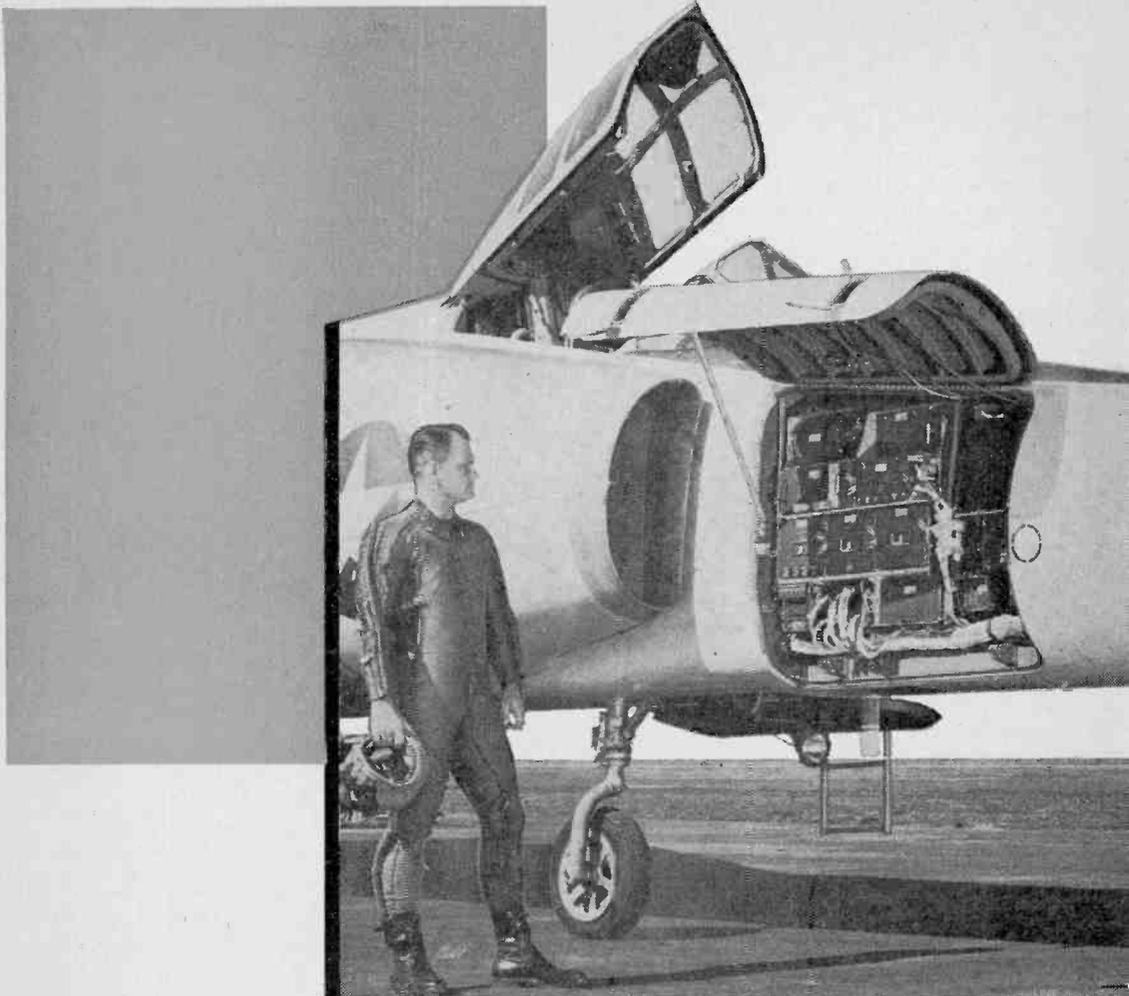
**Digital computers** tend to be large, but some have been put in small packages, as in this Hughes Aircraft model in the fighter plane above. At left, above, two forms of basic computers are shown being examined; the abacus is actually a digital computer, while the slide rule is an analog computer.
