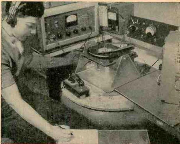
**A permanent record** of test figures of wow, flutter and rumble is kept on all changers. Meter at left measures wow directly in percentages. Flutter is checked on same equipment. Meter at right measures rumble, rated below audibility on the changer. Operator monitors test record tone with earphones. Finally, dielectric safety test of motor and wiring is made with center meter.
