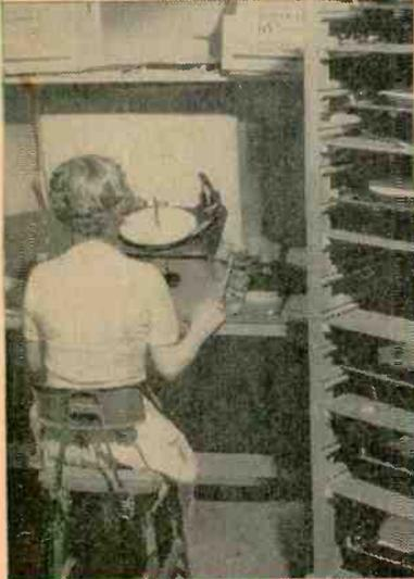
Several changers on rack are checked by quality control operator. If one fails, all get a complete test re-run. Test involves mechanical run-through of all operations, thorough listening with records, amplifier and speaker, and checking for malfunctions or spurious sounds. A rack of tested changers moves on to final packing and the shipping room.
