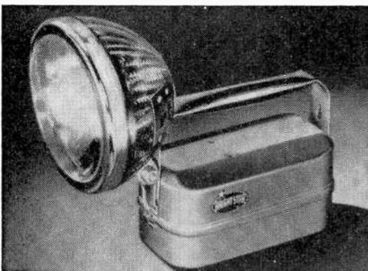
In the center is a new Bright Star sealed beam flasher lantern which is ideal for boating use. It has a 100-hour sealed beam bulb in a specially designed searchlight head that provides a red rear light for both steady glow and red flashing warning. Power source is a 6-volt lantern battery, which clips in quickly.
