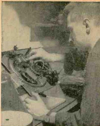
**Start of test procedure** consists of a visual check and final settings of parts fits and clearances. Changer is mounted on special "flip-over" test stand. The tester sets height of tone arm, checks smooth operation of pivots, and adjusts velocity trip friction so that change cycle actuates only after the last groove of the record. Also, stylus pressure is set for all changers.
