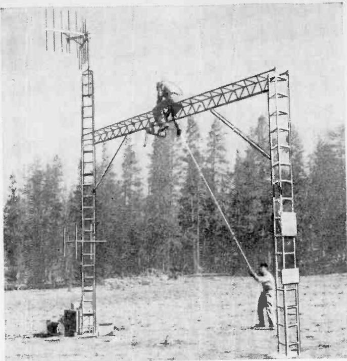
**E**LECTRONICS and radioactive cobalt 60 have joined in the fight to cut flood loss. They are teamed up in radioisotope snow gauges to give weathermen density measurements of the snow pack in remote areas—information used in forecasting spring run-offs.
