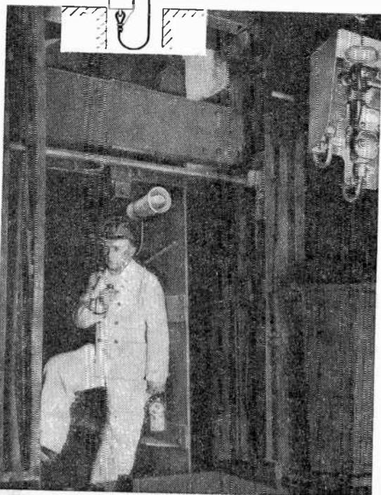
**T**O ELIMINATE the expense and possible failure of an ordinary telephone communications system between a mine head and shaft, a German engineering firm, Standard Elektrik of Stuttgart, has switched to a new method using the elevator hoisting cable as the secondary "winding" of a transformer.
