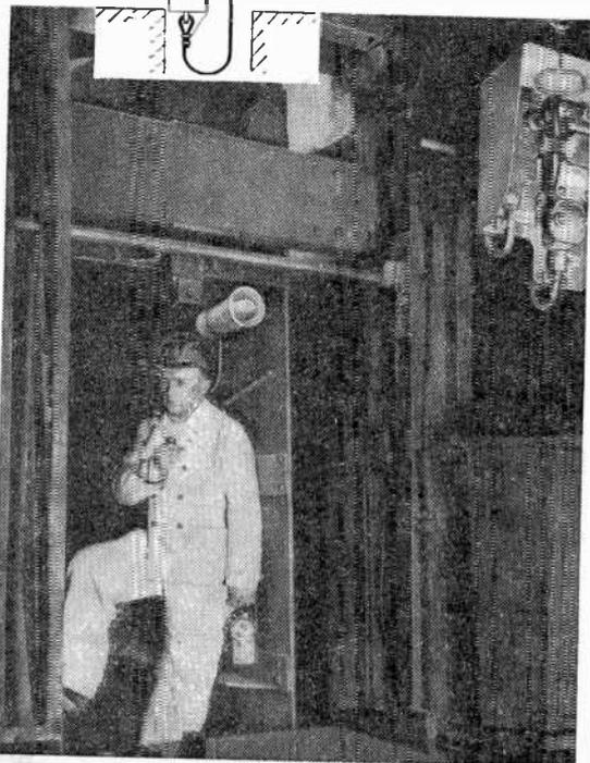
which is electromagnetically coupled to the elevator cable. See top photo. A corresponding voltage is induced in the cable (secondary) which feeds a transistorized loudspeaker system in the car in the shaft, as shown in the bottom photo.
