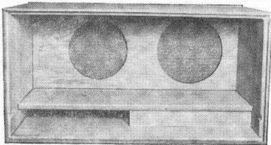
**Internal view** at left shows enclosure just prior to the installation of the loudspeakers. The design of the interior helps to "load" the woofer and provide optimum low-range performance.
