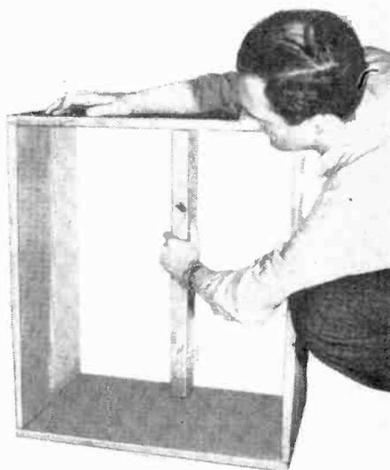
**2** Rear 2" x 4" brace is placed with narrow side flush with rear edge of top and bottom panels. Two #8 flat-head wood screws and glue should be used at each end to hold 2" x 4" brace in position.
