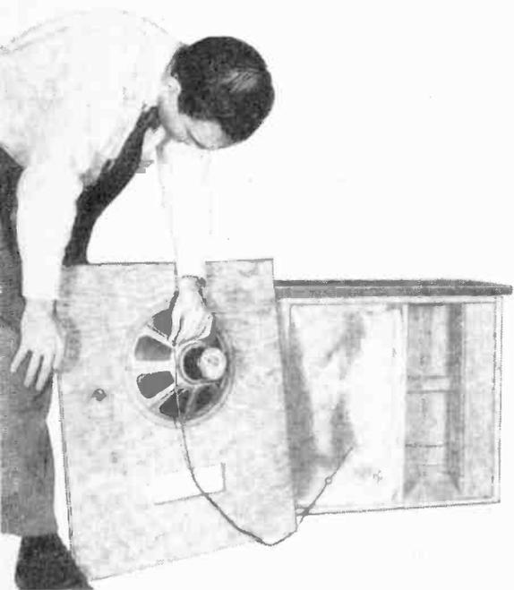
**6** Speaker is mounted on front panel with four  $1\frac{1}{2}$ " bolts and nuts. Speaker cable is attached to the binding posts on the speaker frame and comes out through a small hole drilled in the back panel of the enclosure.
