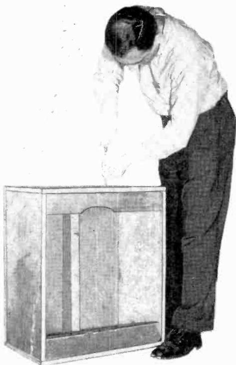
**3** After back panel is glued and nailed in place, 2" x 4" cross-braces are installed. Wood screws and glue are used to tighten rear panel to the 2" x 4" rear brace and to secure cross-braces. Cracks should be caulked with wood putty to prevent air leaks.
