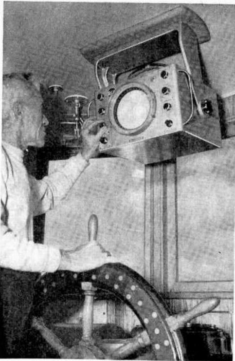
**Ceiling radar installation** saves space and allows shorter lead-in cables to antenna atop wheelhouse. (RCA photo)
