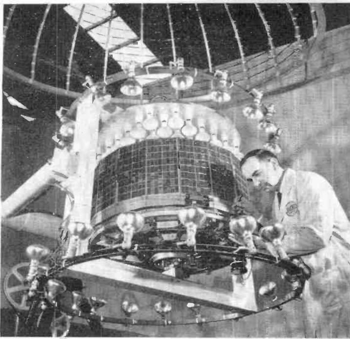
Magnetic orientation system being tested at RCA's Space Center in Princeton, N. J. Lights above and around the satellite are used to check operation of solar cells which surround satellite.
