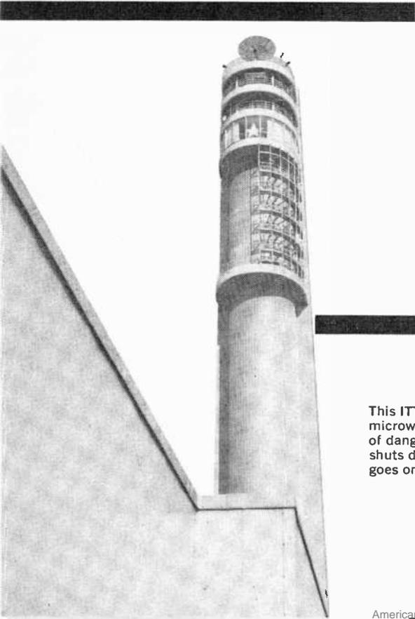
This ITT tower in Nutley, N. J., is used for microwave experiments. To prevent the possibility of dangerous radiation, a trapdoor interlock shuts down the transmitters whenever a technician goes on the roof to service the antennas.
