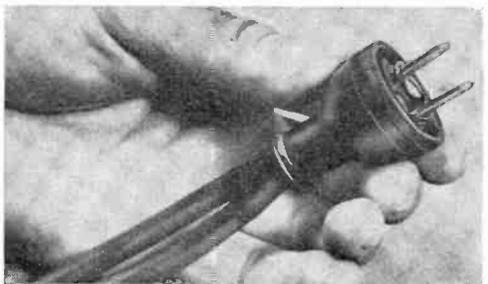
sulting doubled-up power cord will safely carry up to 1200 watts. However, be sure not to overload your power outlets.
