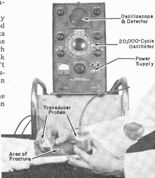
The soniscope in action—checking the healing of a broken leg. Ultrasonic sound waves pass between two transducer probes; the speed of the waves is displayed on an oscilloscope.
