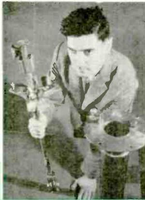
Hughes' maser microwave amplifier has ruby and magnet at bottom. Unit is installed in coolant container (above, right) to supercool ruby near absolute zero.
