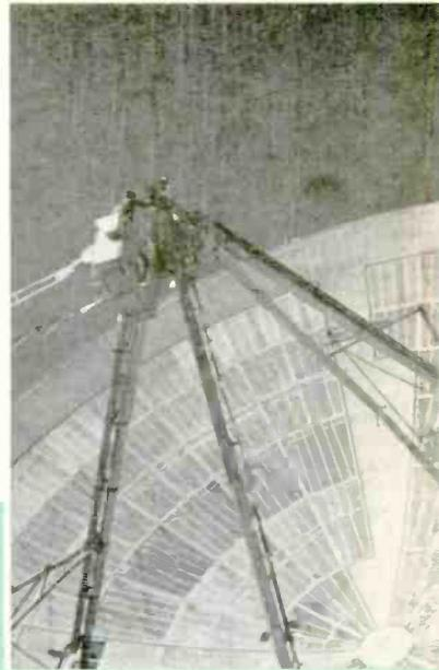
NASA parabolic antenna catches fleeting signals from space; they're amplified by supercooled ruby maser mounted in front.
