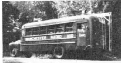
Once operated as an army bus, this vehicle is now known as KBC8000. It was converted into a mobile communications center by members of Manchester Radio Aid, Inc. Equipped with four transceivers, a p.a. amplifier, and living facilities for a two-man crew, it's ready to go at a moment's notice.
