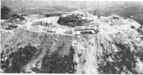
**T**HE ENTIRE top of a mountain at Ajangote in Ghana, Africa, has been "decapitated" to make room for a high tower designed to support TV transmitting antennas, and buildings to house transmitting equipment. The elevation
