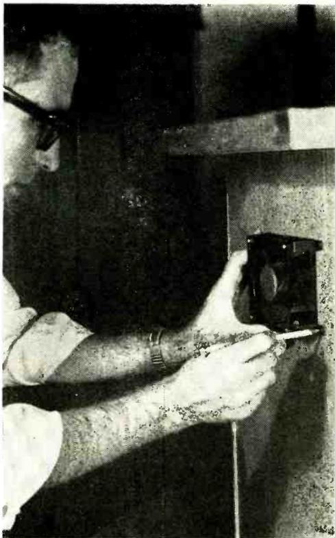
Spot selected to mount the Whisper fan should permit free air flow. Mark off the four mounting holes and cut the opening with a sabre or keyhole saw.
