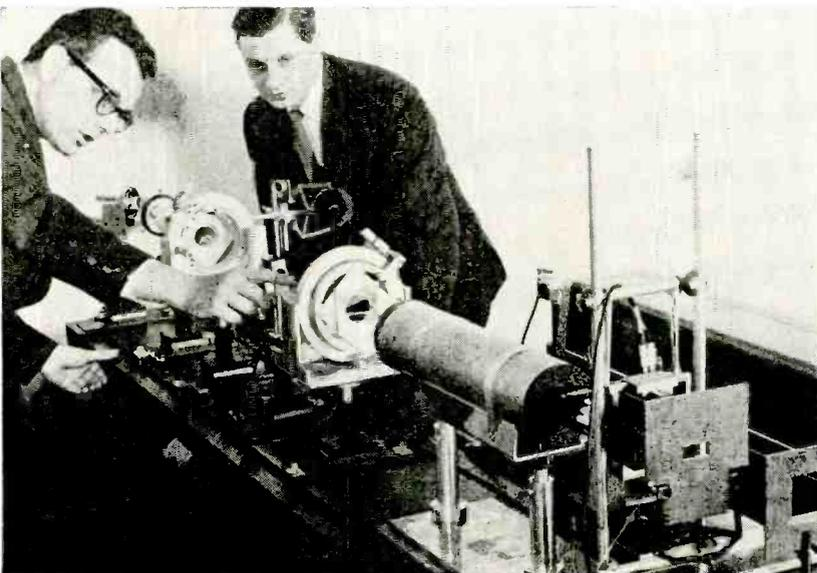
RED AND BLACK TV—An ultrasonic diffraction cell that directs acoustic waves of varying frequency to deflect a laser beam across a screen has been developed by Zenith Radio Corp. Other cells provide intensity modulation and vertical deflection, performing the same jobs as picture tubes and deflection yokes in conventional TV sets. Because the helium-neon laser emits a red light beam, the picture on the screen is red and black in this experimental television picture display system.
