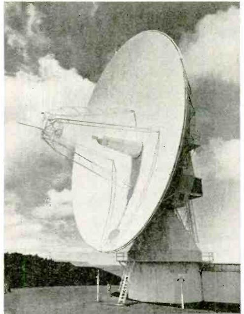
TALLER THAN A TEN-STORY BUILDING—Six foot saucer-shaped antennas will be used to align two huge 85'-diameter antennas with sharpshooter precision at "boresight" test ranges being readied in Washington and Hawaii by General Telephone and Electronics Corp. The 135-ton antennas will be used for satellite communications.
