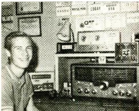
Steve Buerg, WN6THT, Daly City, Calif., made 458 contacts in 46 states and five continents in two months. How's that for a record? A Hallcrafters HT-40 transmitter and SX-101 receiver and a Hy-Gain 14-AVS vertical antenna are his tools.
