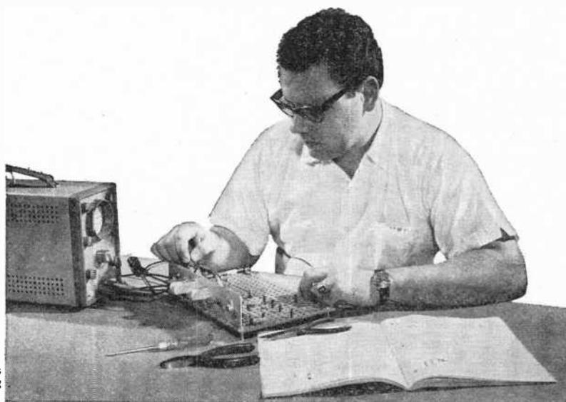
Performing transistor experiments on programmed breadboard—using oscilloscope
