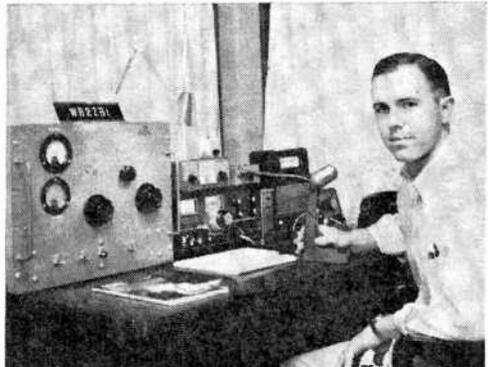
Tom Massey, WB2ZBI, Glen Rock, N.J., has worked all states and 85 countries. A Swan 500C transceiver drives a homebrew linear amplifier to feed a Mosley TA-33 beam or a doublet antenna. He operates SSB and CW but says he prefers the latter.
