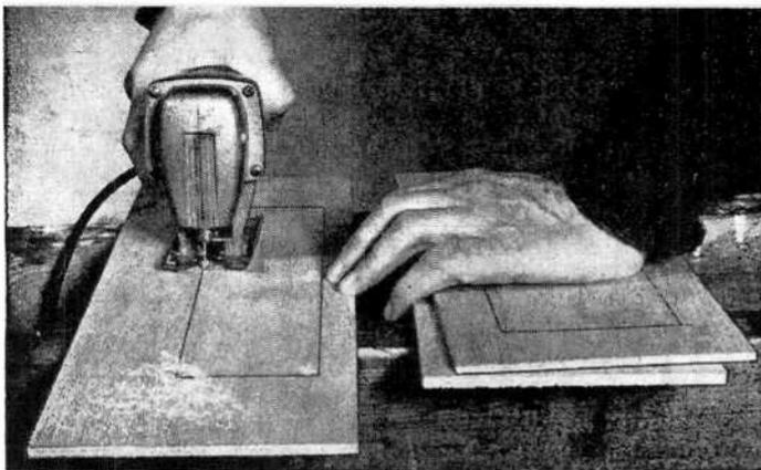
Sabre saw is best for making cutouts in thin plywood. If sabre saw is not handy, carefully use crosscut keyhole saw.
