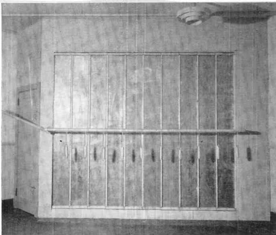
With filter in position shown here, frequency components above 5000 Hz were eliminated. The lever at left controlled filter louvers to permit quick changes in frequency response.
