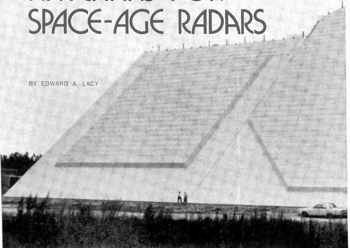
functioning for quite a while now. The biggest one, the AN/FPS-85, (below) located at Eglin Air Force Base, was designed to meet the need for space tracking. Built by Bendix Corp., the radar is housed in a wedge-shaped building the size of a football field. Seen from either end, the building has the shape of a right triangle. Its sloping roof contains the individual transmitting and receiving modules. Head-on, the building looks more like a giant billboard instead of a radar installation.
