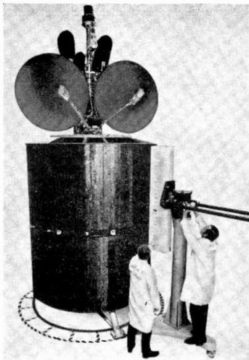
Intelsat IV satellite is shown here being tested in Hughes r-f laboratory.
