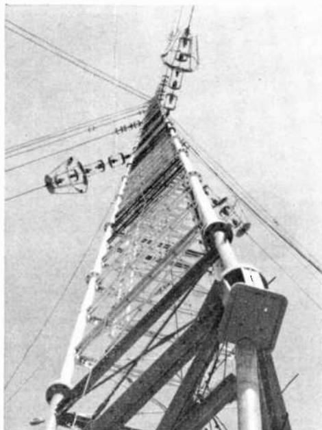
The towers are painted with alternate bands of orange and white to provide aircraft warning, though it is said that the steel's use would be enhanced if it were permitted to oxidize and form its own protective coating. ◆
