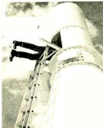
*Difficult position is required of technician shown here working on the bearings of a TACAN rotating antenna assembly.*
