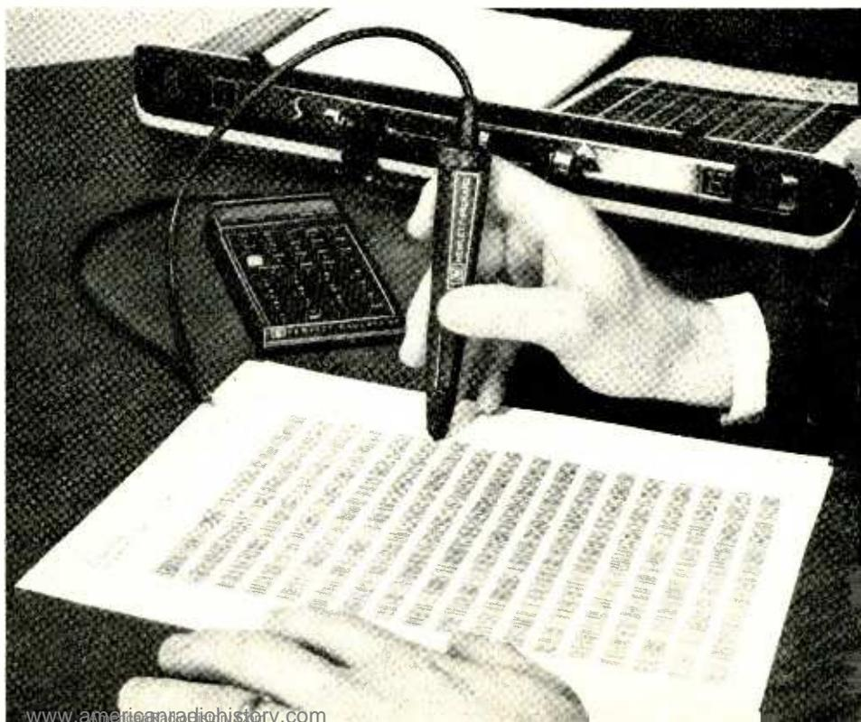
Programs and data can be loaded into the HP-41 via the keyboard or with the help of a handheld wand that reads bar code. The wand permits lengthy listings to be loaded quickly and *error free*. Barcode listings are supplied with HP-41 software. A service for converting commonly used programs into bar code is available.
