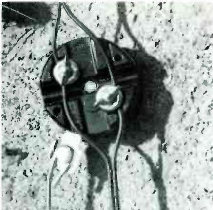
An antenna-discharge unit helps to protect against equipment damage caused by induced voltage during lightning storms. But don't rely on it to protect against a direct lightning strike. And never ever use the system during electrical storms.
