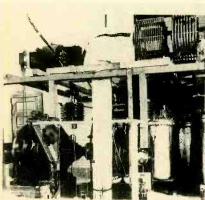
*This was the most powerful rotary spark-gap transmitter of its time. Installed at a Navy radio station, it produced 100 kW on a frequency of 113 kHz. In the lower portion of the picture are the motor and rotary spark gap. To the lower right are the compressed-air high-voltage capacitors, and on top of the platform you can see the oscillation transformer.*
