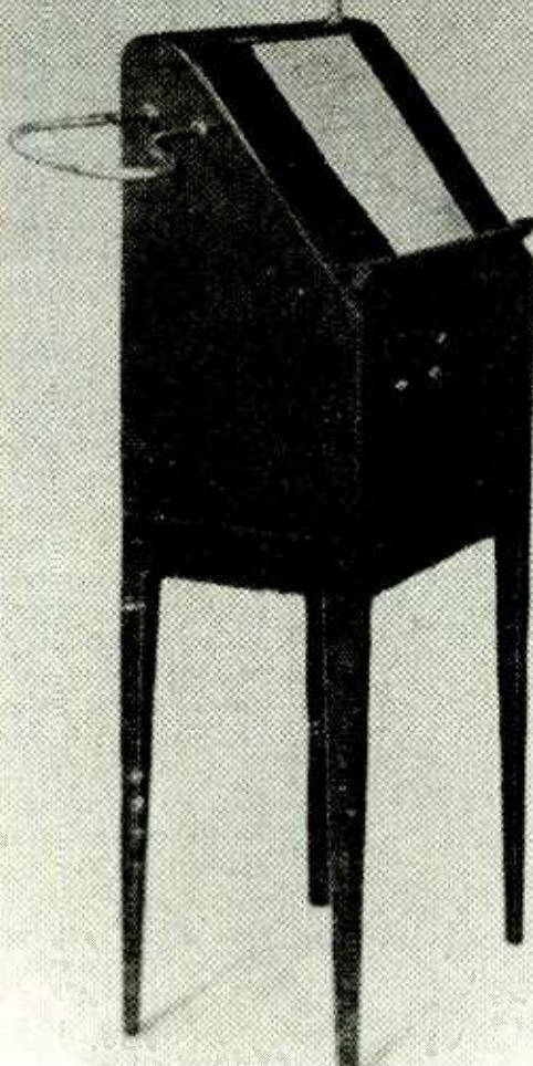
A photo of the Theremin taken from RCA advertising literature. The straight rod controls pitch while the loop controls volume.
