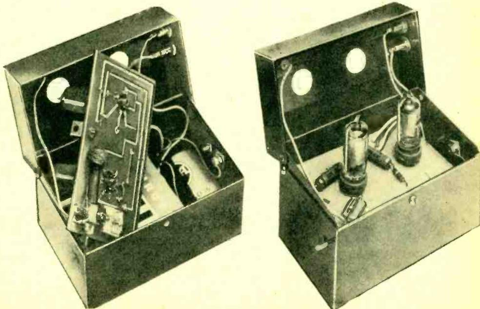
The photos above show completed receiver with cabinet open. At left is view of printed circuit board being put into place. Photo at right shows completed assembly. Note location of phone jacks, batteries, etc.
