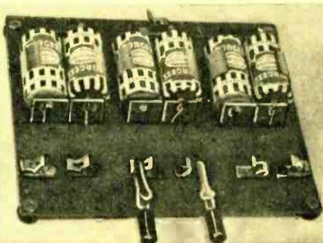
"tap" into the individual battery boxes, obtaining nominal output voltages covering the range of 1.5, 3, 4.5, 6, 7.5 and 9 volts.
