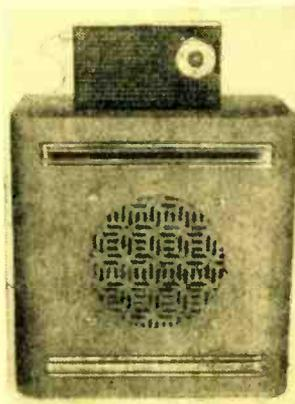
"Picnic PowerAmp" is shown in photo above ready for operation. The pocket receiver is placed on the amp, and the input for the amp is taken from the headphone jack output of the pocket receiver.
