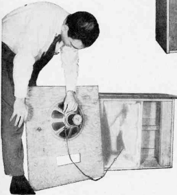
5 Finishing panel, although not necessary, may be added for the sake of appearance. Four wood screws through cabinet hold 30" x 16" panel in place. Interior of top compartment should be loosely lined with Fiberglas, rock wool, or other acoustical damping material. Cabinet may be used upright as lowboy, finished or unfinished, as desired.
