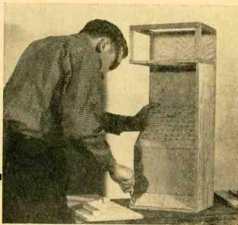
Side view of enclosure, showing its perforated resistive panel. All joints are screwed and glued.
