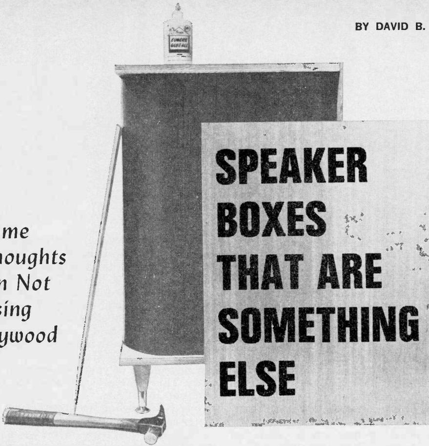
**W**HETHER by design, accident, or habit, plywood has become the common working material of hi-fi enthusiasts who build their own speaker enclosures. Considering that plywood is stronger than solid lumber of equal thickness and that it is available in large, flat sheets, it is not a bad choice.
