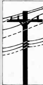
SECONDARY DISTRIBUTION LINES (115/230V) 0.1-1μT, WITH A SLOW MAGNETIC FIELD DROP-OFF OF 1/r (DUE TO UNBALANCED PHASE AND NEUTRAL LINES)
