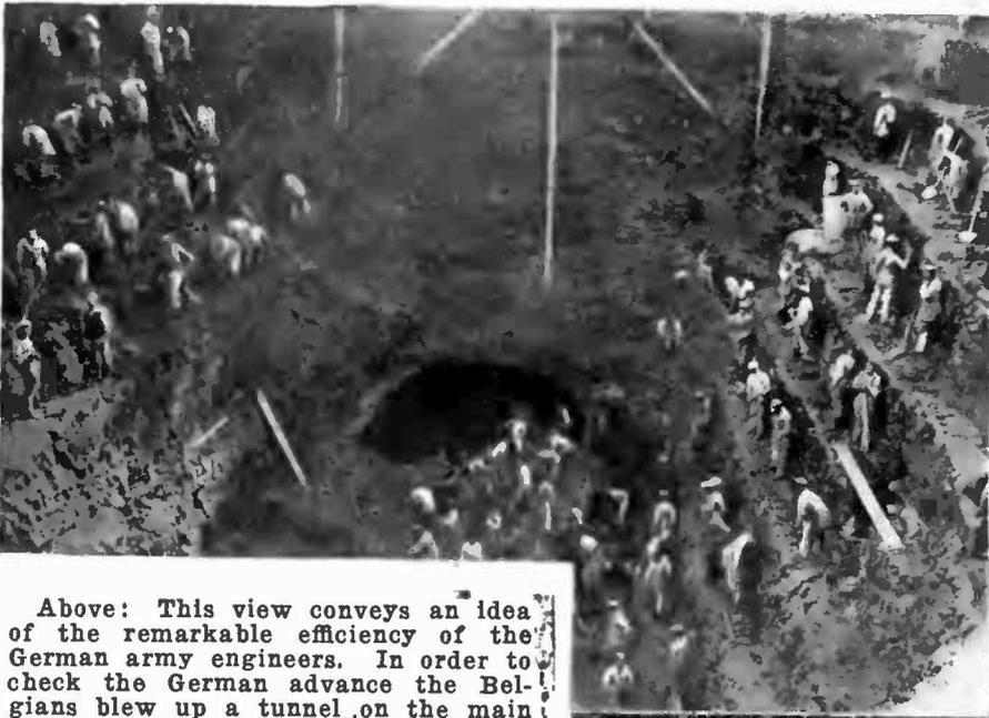
Above: This view conveys an idea of the remarkable efficiency of the German army engineers. In order to check the German advance the Belgians blew up a tunnel on the main line of a railroad. Here are seen the German engineers excavating the ruin.
