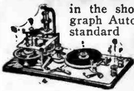
in the shortest possible time. The Omnigraph Automatic Transmitter combined with standard key and sounder. Sends you telegraph messages at any speed just as an expert operator would. Five styles, \$2 up; circular free. **OMNIGRAPH MFG. CO.**
