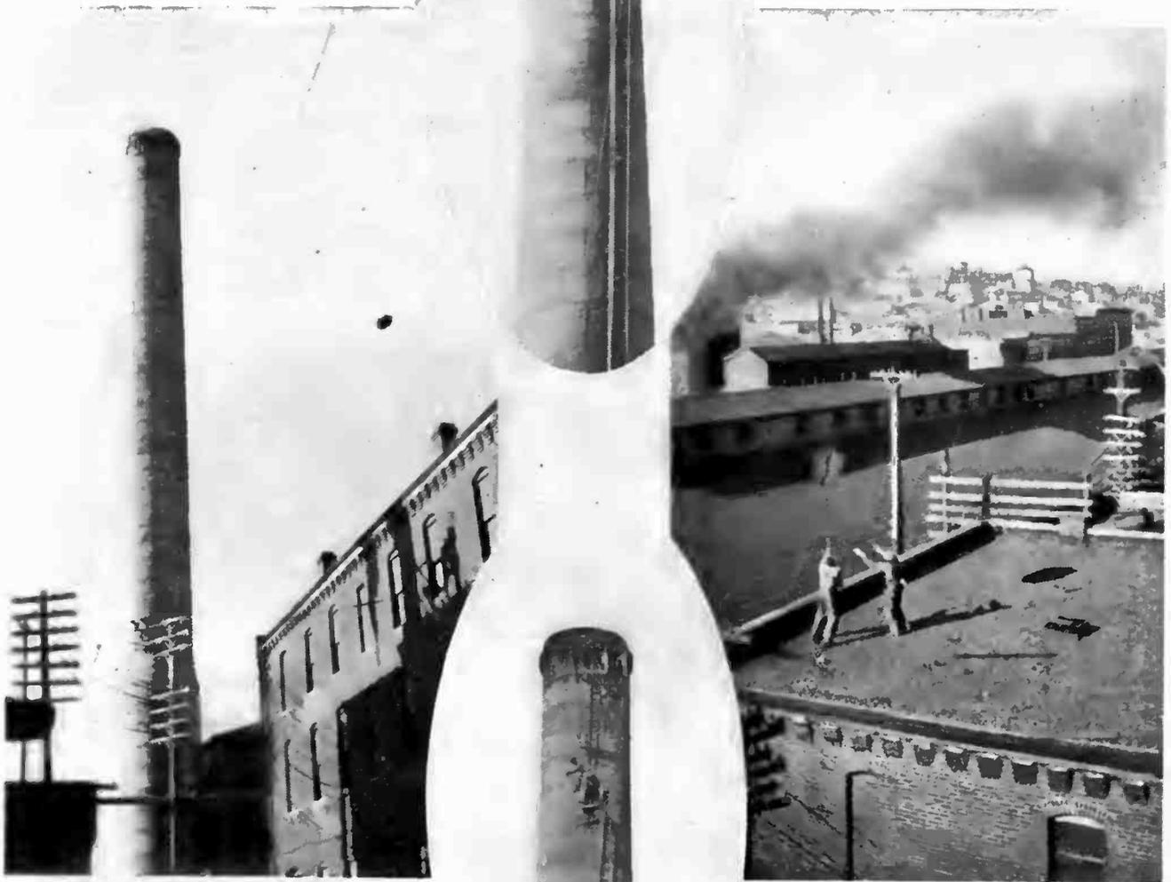
In order to carry the initial string to the top of a tall chimney, a rather novel method was employed. The string was fastened to an umbrella that was placed in the stack so as to be pushed upwards by the heated gases. The
