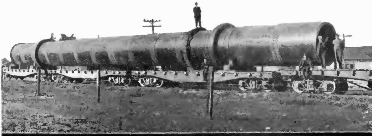
Four Cars Were Required to Haul this Steel Tube Measuring 120 Feet in Length and Weighing 149,000 Pounds.
