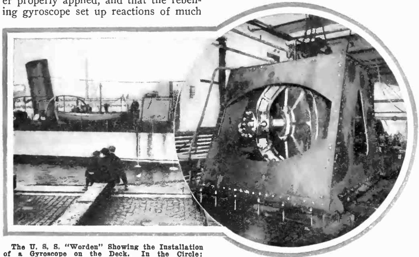
The U. S. S. "Worden" Showing the Installation of a Gyroscope on the Deck. In the Circle: Method of Mounting a Gyroscope on Shipboard.
