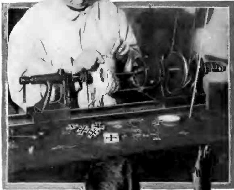
Woman worker polishing the finished Iron Cross on a buffing wheel. Below: An expert workman engraving an Iron Cross.
