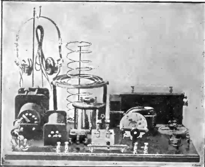
Receives up to 2600 miles. Sends up to 60 miles. Consists of 1/2 kilowatt vibrator transformer, Rotary Spark Gap, new type oscillation transformer, variable condenser, loose coupler and loading coil —tunes up to 3300 meters — detector, buzzer test and potentiometer. Complete in every detail ready to work.
