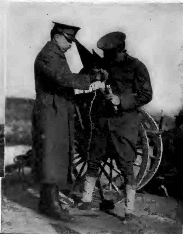
At the right: Preparing a charge of the new explosive, TrotoI-Gelatine, for the tests on land and submarine mines at Fort Wadsworth, S. I.
