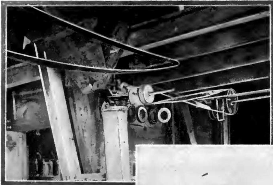
To the left: Interior of the windmill building showing arrangement of bevel gears at the base of the windmill shaft. By means of these gears the power is transmitted to a horizontal shaft.
