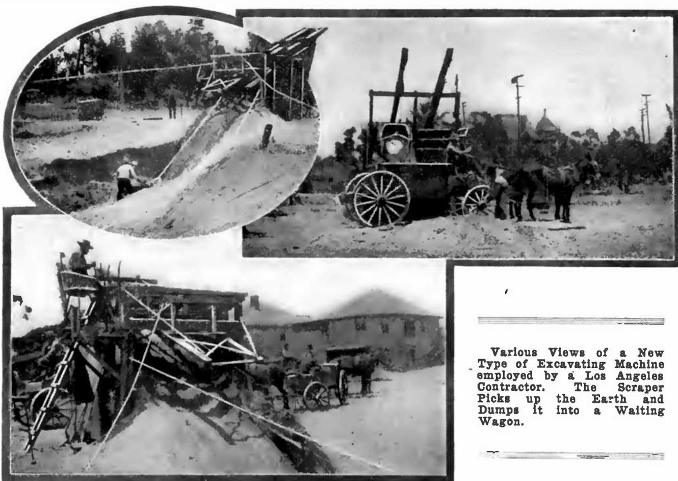
Various Views of a New Type of Excavating Machine employed by a Los Angeles Contractor. The Scraper Picks up the Earth and Dumps it into a Waiting Wagon.
