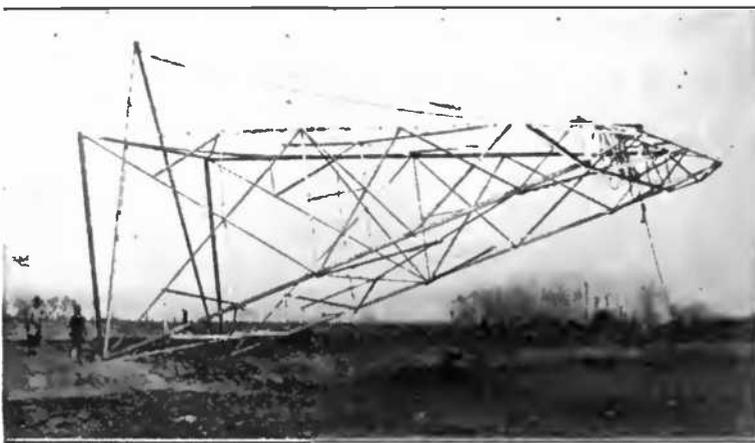
Eight or More Horses are Required to Erect a Steel Tower for Electric Cables.
