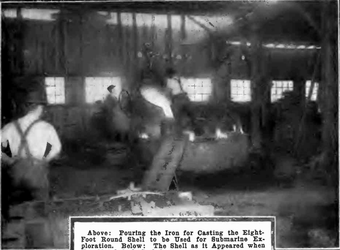
Above: Pouring the Iron for Casting the Eight-Foot Round Shell to be Used for Submarine Exploration. Below: The Shell as it Appeared when the Metal had Cooled.
