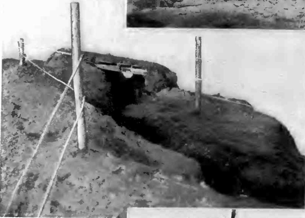
A section of the English coast trenches. These earthworks are constructed along the same lines as those on the Continent, and are provided with bomb-proof shelters and barbed wire entanglements. They are intended to withstand a bombardment by warships and repulse an attempted landing.
