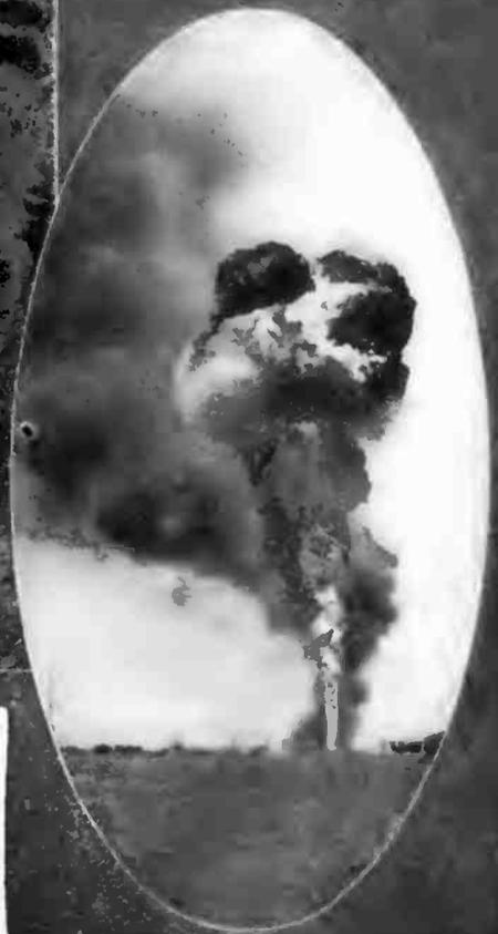
At the Right: A gusher in the oil fields near Bakersfield, Calif., recently caught fire and burned for several days before it could be extinguished. Eighty acres of ground was burned over and the huge torch was only extinguished after several days' effort, using metal plates and live steam.
