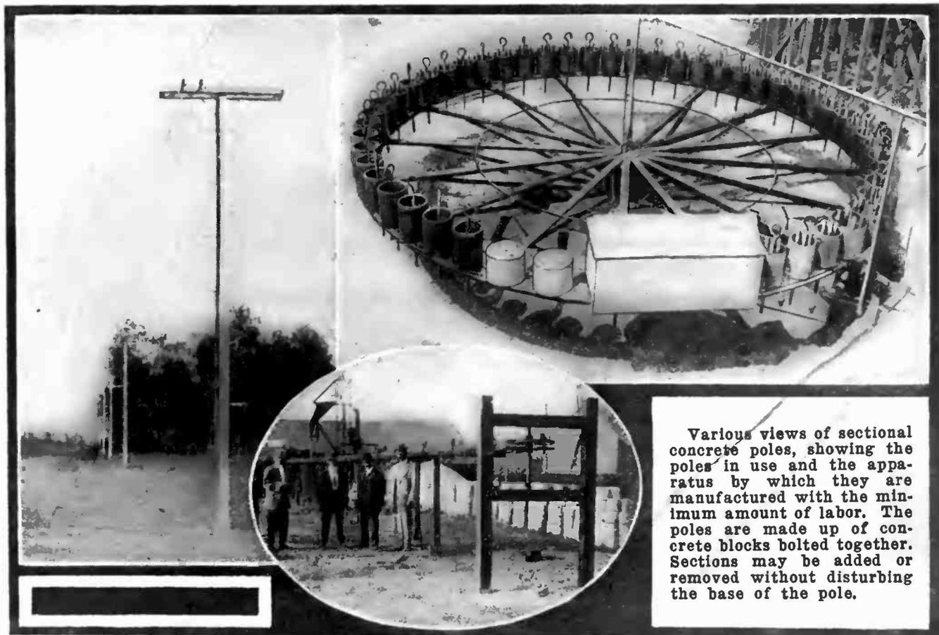
Various views of sectional concrete poles, showing the poles in use and the apparatus by which they are manufactured with the minimum amount of labor. The poles are made up of concrete blocks bolted together. Sections may be added or removed without disturbing the base of the pole.
