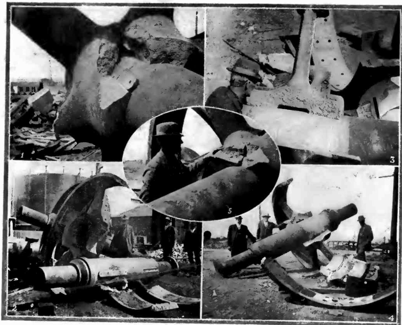
(1)—What an ineffectual discharge of dynamite did to the hub of a big steel wheel. (2)—Another view of the same wheel after being shattered by the dynamite discharge placed at the hub. (3)—Remarkable straight fracture of the cast steel wheel at the hub, caused on the opposite side to where the dynamite was inserted. (4)—Another view of the steel wheel and its shaft. (5)—An unsuccessful attempt to shatter the wheel by a dynamite blast.
