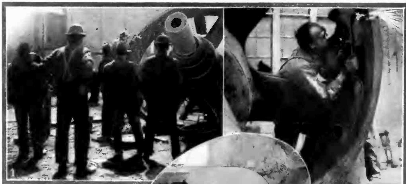
(1)—Watching a skilled operator cut through the four-inch rim of a huge cast steel wheel. (3) — Four sticks of dynamite inserted and discharged in this cast steel cylinder achieved the result shown.
