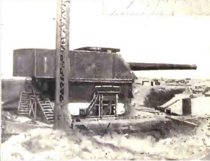
A fourteen-inch gun installed in a land turret at the Sandy Hook proving grounds where the turret is being thoroughly tested. The idea of using a turret for land guns is not a new one, but it promises to give greater combative power to coast defenses.
