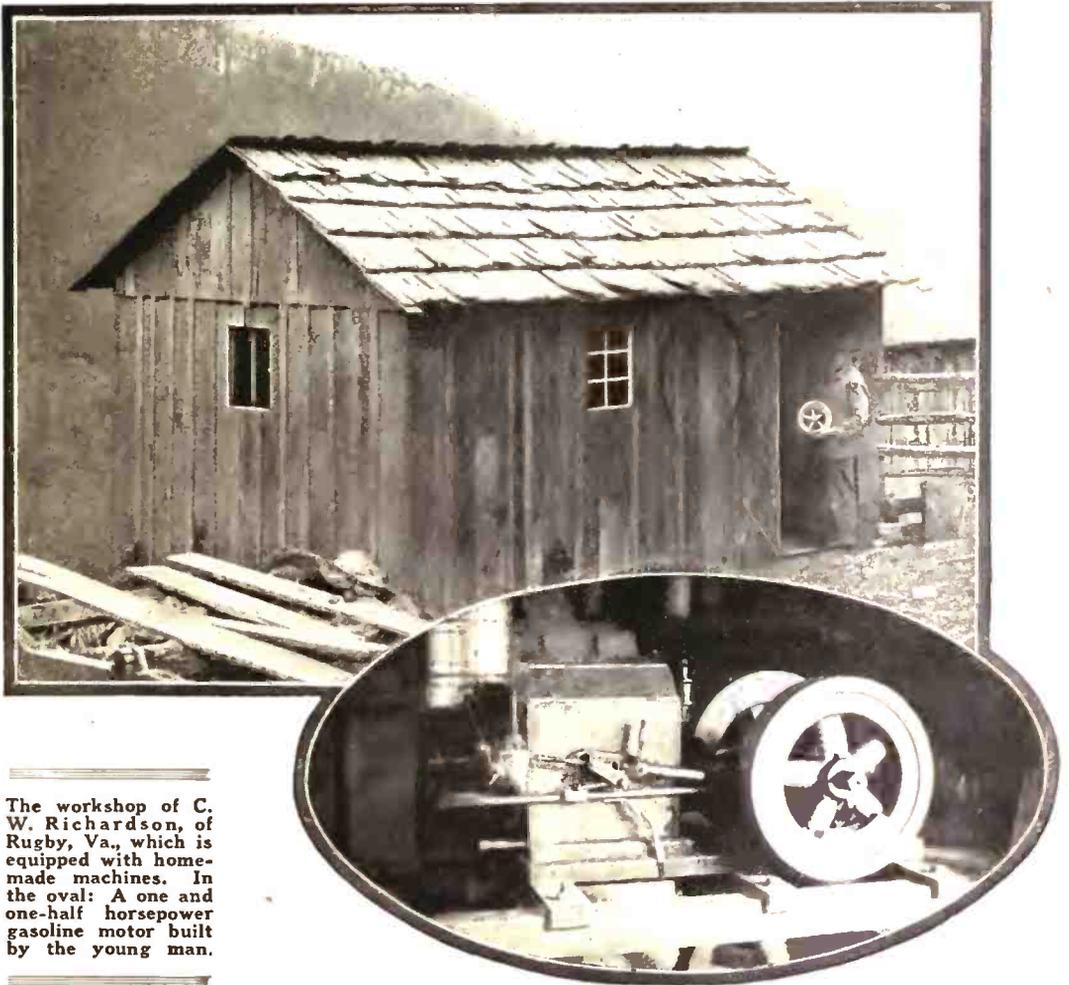
The workshop of C. W. Richardson, of Rugby, Va., which is equipped with home-made machines. In the oval: A one and one-half horsepower gasoline motor built by the young man.
