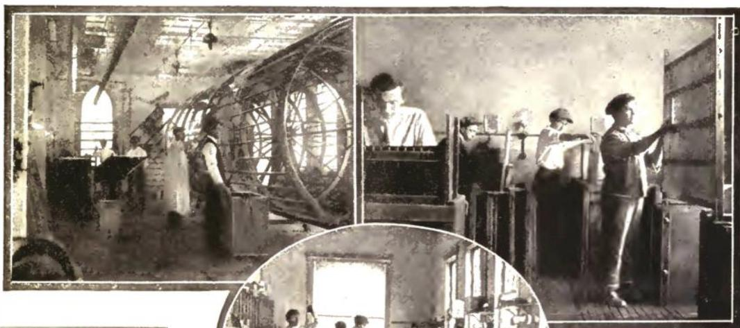
Above: A Drying Room in Which the Wet Films Are Dried on Wooden Drums. In the Oval: The Inspecting Room—One Corner of the Systematized Solax Finishing Plant.
