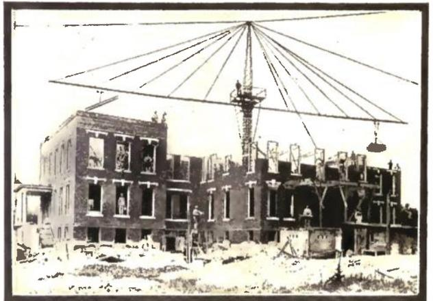
A School Building Being Erected with the Aid of a Revolving Crane Mast. Much Time and Labor are Saved by the Use of this Equipment.
