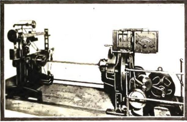
A Machine for Testing Strength of Steel, which has a Capacity of 230,000 Inch Pounds.
