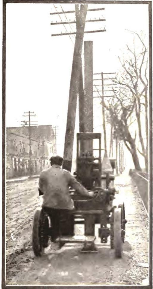
The Gasoline-Operated Tamping Machine is a Recent Addition to the Ranks of Labor-Saving Devices. It Does the Work of Several Men.
