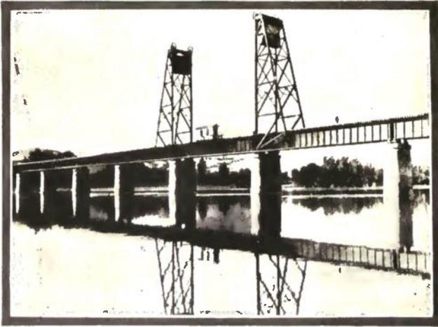
The Lifting Power of this Deck Girder Bridge is Furnished by a Gasoline Engine.
