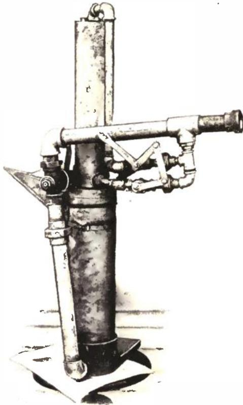
By Means of This Device it is Possible to Inject Ballast Under Railroad Ties After the Track has been Lifted.
