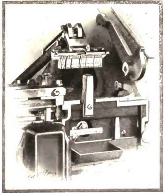
The Elevator Arm in the Act of Taking a Line of Matrices which are to be Carried to the Distributing Mechanism.
