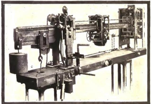
A Scale in which Electricity Does all the Work, Both Automatically Weighing Truck Loads and Keeping a Permanent Record.
