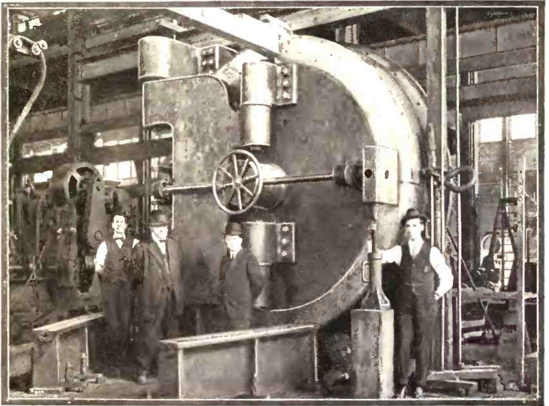
The Largest Circular Vault Door and Vestibule Ever Constructed, on the Floor of the Factory, Ready for Shipment. So Wonderfully Balanced is the Huge Door that it May be Swung Open by Hand.
