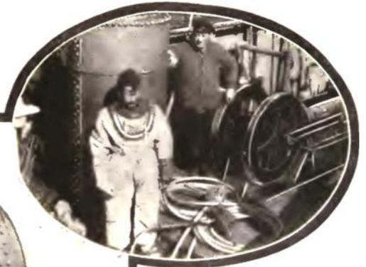
The Experimental Chamber in which Drs. Leonard, Hill and Greenwood Underwent Air Pressures Slightly in Excess of that in a Diving Suit at a Depth of 210 Feet. In the Oval: A Steam-Driven Air Compressor Charging the Reserve Tank from which the Diver is Supplied with Air.
