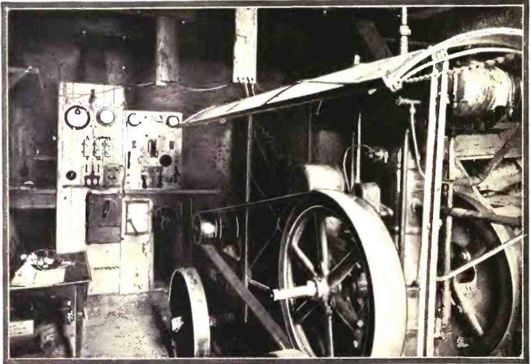
The German Army is Using this Type of Electric Generating Plant Mounted on Wheels and which can be Immediately Installed at Any Desired Point for Supplying Current for Illumination and Other Purposes.
