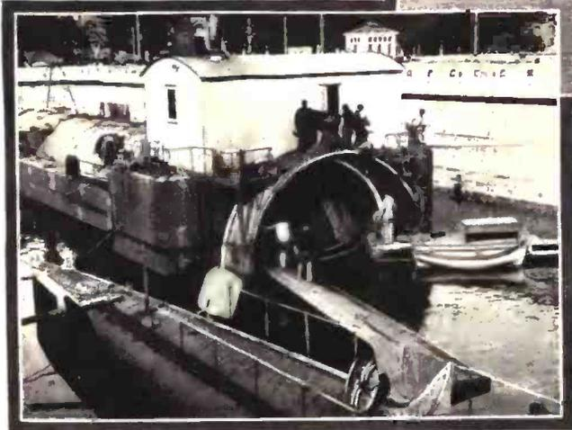
Above: The Launching of the Italian Testing Dock for Submarines, at the Fiat-San-Giorgio Shipyards Near Spezia. The Testing Dock Consists Essentially of a Big Tube Made of High Tensile Steel, Permanently Sealed at One End and Closed at the Other by Means of a Globular Caisson. At the Left: Entrance to the Testing Dock.
