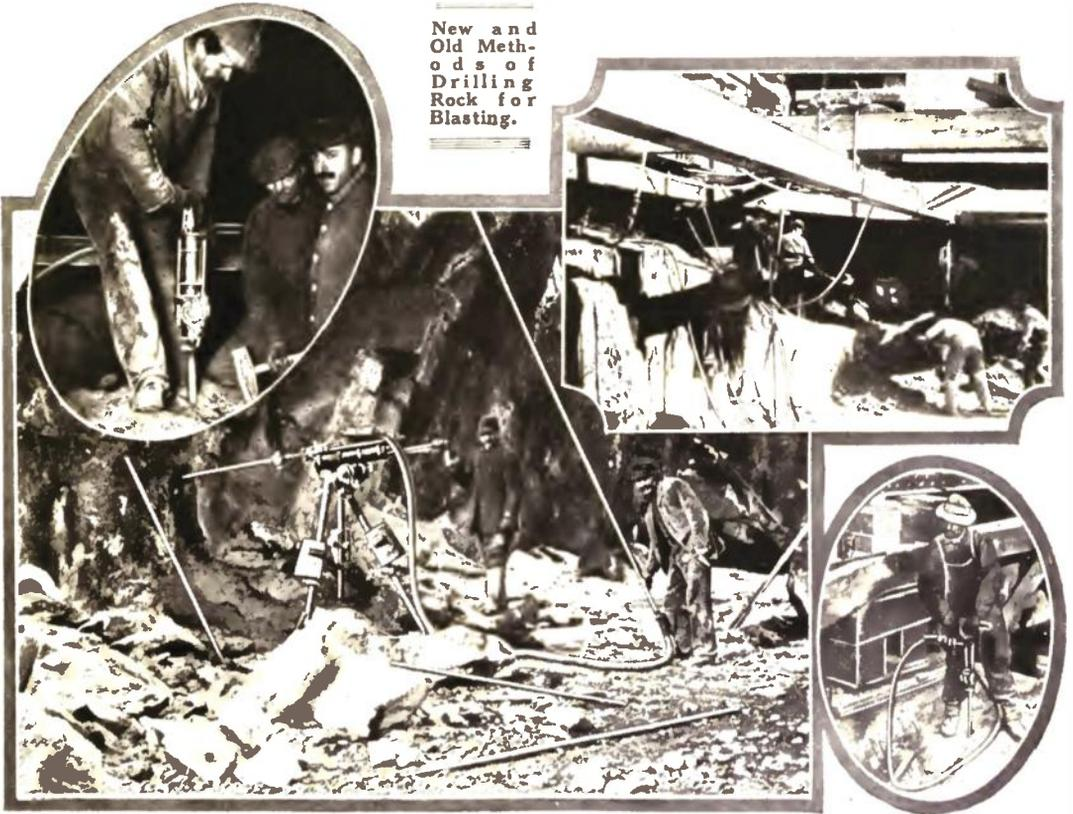
heavy iron tripods. Weight was the predominating factor—the apparatus was heavy and the blow was heavy, but the speed of operation was correspondingly slow; in fact, the apparatus was so cumbersome that it frequently required as much time to set up the drill as to drill the blast hole.
