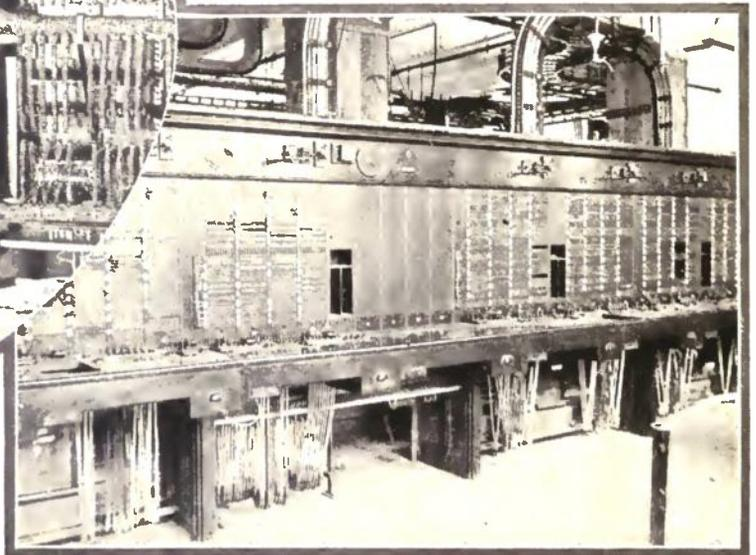
tance exchange at Los Angeles, Cal. Any line, inside or outside of the exchange, may be plugged into the board for any kind of test imaginable. Breaks or crosses on long lines are measured to a fraction of a mile with a Wheatstone bridge and galvanometer. A line inside the exchange causing trouble is cut off
