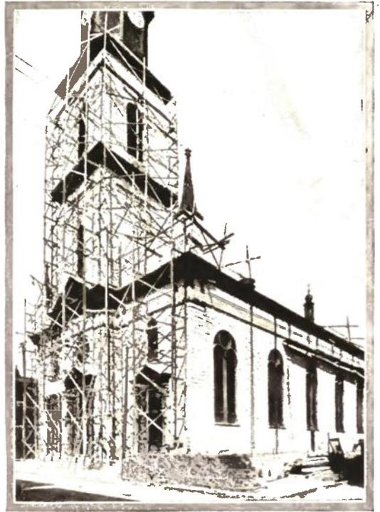
Thin Slabs of Concrete Placed Over the Brick Walls of this Church have Given it the Appearance of a New Building.
