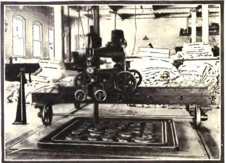
By Means of an Intricate Cog Track on the Floor, this Sewing Machine is Guided in Sewing Comforter Layers Together.
