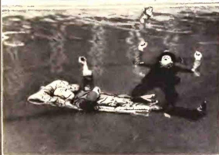
Two men floating in the water, due to the buoyancy of Kapok. One of them is resting on a blanket of carded Kapok measuring five feet by two feet six inches and which will keep any person afloat for an indefinite length of time. The other man is wearing a Kapok padded suit.
