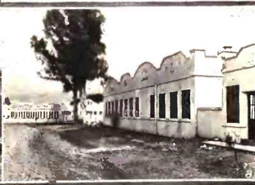
appearance. The smaller buildings, which are used for picture producing purposes only, are simple front exteriors which are erected in a day and are torn down just as soon as they have served
