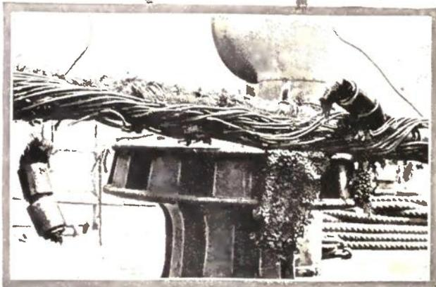
the terebo are repulsed with a thin sheathing of brass. A more inert but none the less virulent enemy is the chemical iodine, which is a by-product formed in the maturation of sea-weed. Iodine rapidly corrodes the armoring wires of the cable.
