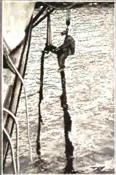
Above: Grappling for a Cable at Close Quarters. As May be Seen in this View, the Cable Ships are Often Obligated to Operate Very Close to the Shore. At the Right: Hooking an Ocean Cable in Order that Repairs May be Made. In the Oval Below: Crew of the "Mackay-Bennett" Breaking Away Ice from the Forecastle.
