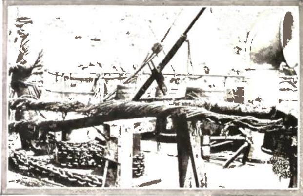
Above: A Section of an Ocean Cable on the Deck of the "Makay-Bennett," Ready to be Repaired. Below: Another Near View of an Ocean Cable, Showing How Damaged the Covering May Become, Especially in the Instance of Cables Near Shore.
