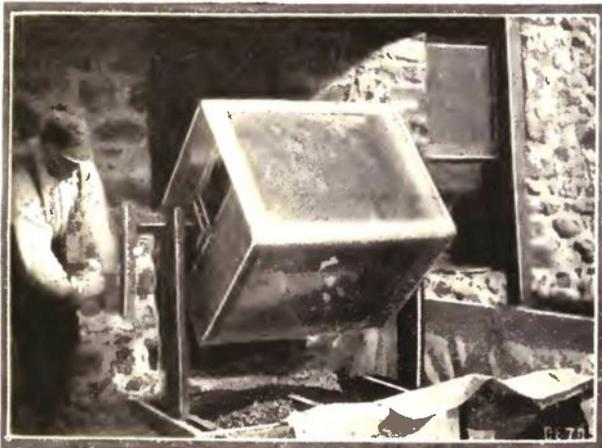
A Simple Screen Arrangement for Separating Seeds of Cone-bearing Trees from Their Cones.
