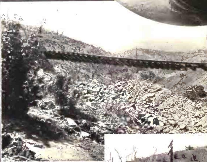
A near view of a washout in northern California and its effect on a railroad track. The rails and wooden ties have been left hanging in the air after the earth beneath them was washed away by a torrent of water.
