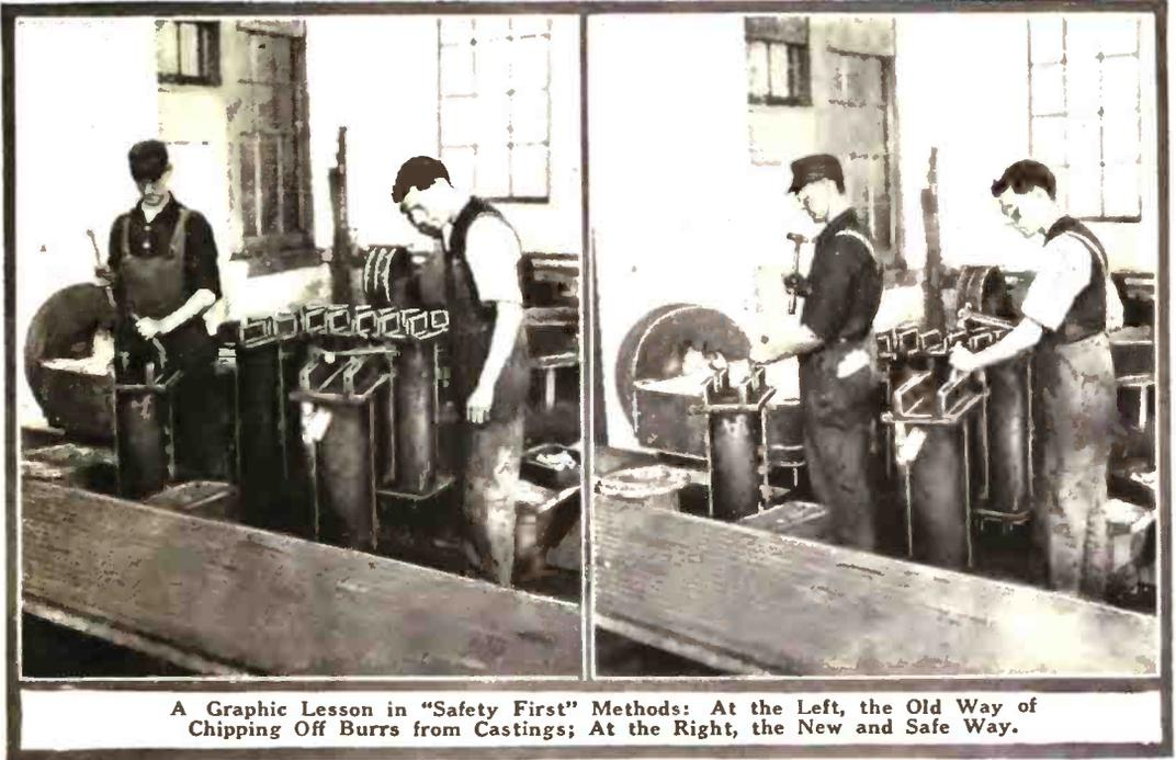
A Graphic Lesson in "Safety First" Methods: At the Left, the Old Way of Chipping Off Burrs from Castings; At the Right, the New and Safe Way.
