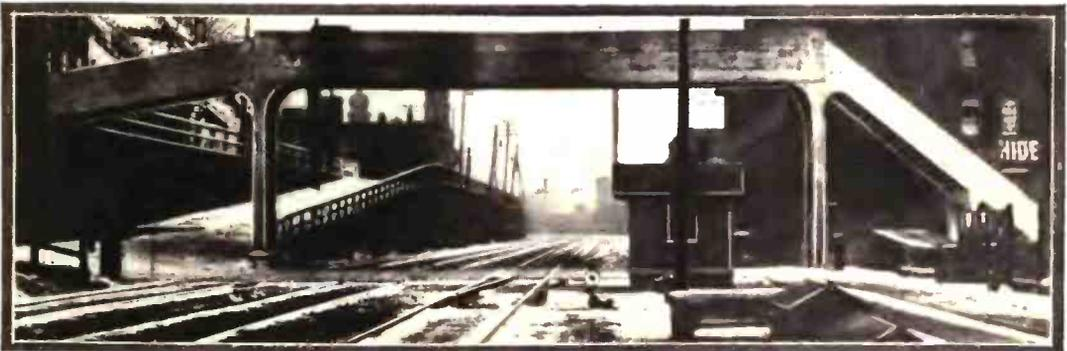
The Same Bridge as Above After it Was Covered Over with Concrete So as to Render it Impervious to the Action of Locomotive Smoke.
