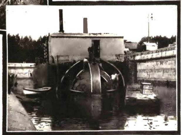
Two Views of the Entrance to the Testing Dock, Showing the Globular Caisson in Place. After a Submarine Has Been Placed in the Testing Compartment, Hydrostatic Pressure is Gradually Increased by Means of Pumps, So as to Submit the Walls of the Under-water Craft to the Same Conditions as if it Were at a Corresponding Depth Below the Surface of the Sea.
