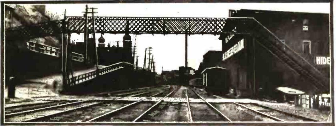
A Typical Iron Bridge Crossing Railroad Tracks, Which Ultimately Became Weakened by the Corrosive Effects of Locomotive Smoke.
