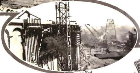
The Entire Structure, with the Exception of the Main River Span, Will be of Reinforced Concrete.
