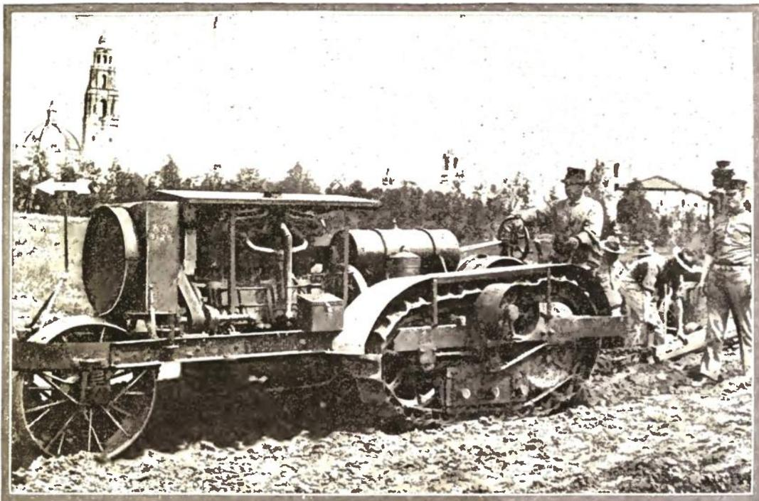
We are told that this is a "Machine War." So it is. Even the trenches of field fortifications, made so that a retreating army may retire to them when hard pressed, are dug by machines. This picture shows the experiment in machine trench digging carried out at the San Diego Exposition. A gasoline farm tractor was used to haul a file of sappers and digging machinery.
