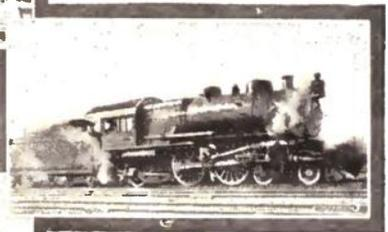
Above: Atlantic Type Locomotive Fitted with Rotary Valves.
