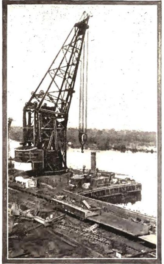
This Gigantic Crane of German Manufacture is Now Being Used for Mounting Guns in the Canal Zone.
