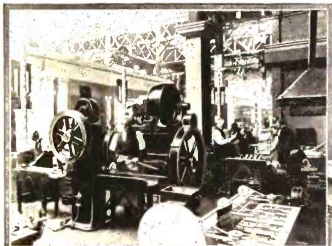
The White Apparatus in the Foreground is the Electrolytic, or Metal Refiner. At the Extreme Right is the Electric Furnace. The Large Machine in the Center is the Rolling Mill.
