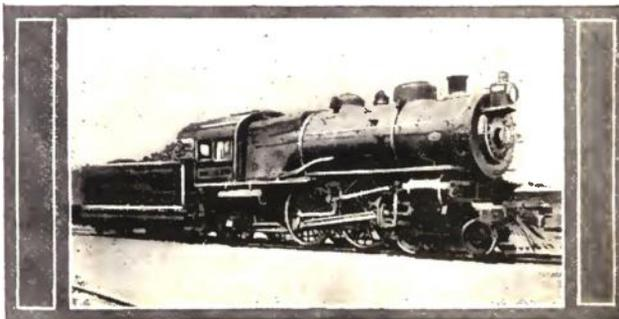
The Third Atlantic Type Locomotive Used Was in Reality a Freight Engine Boiler Mounted on Passenger Engine Wheels.
