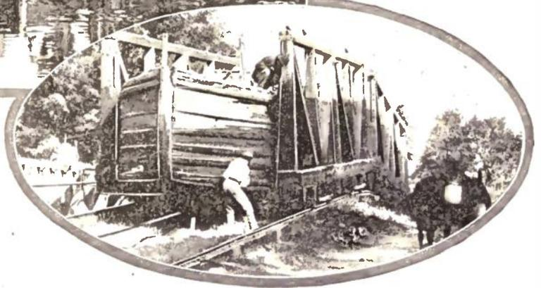
Two Views of a Railway for Carrying Canal Boats Up a Mountain-side. The Canal Boats Float Into a Cradle Mounted on Wheels and Are Then Hauled Up the Incline by Means of a Cable.
