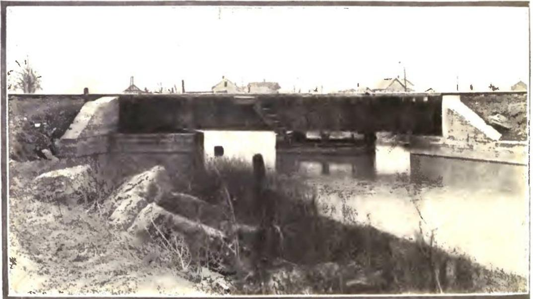
A Drawbridge Which is So Constructed That Trains May Pass Over it at Full Speed. It Requires One Man About Half an Hour to Open and Close the Bridge.
