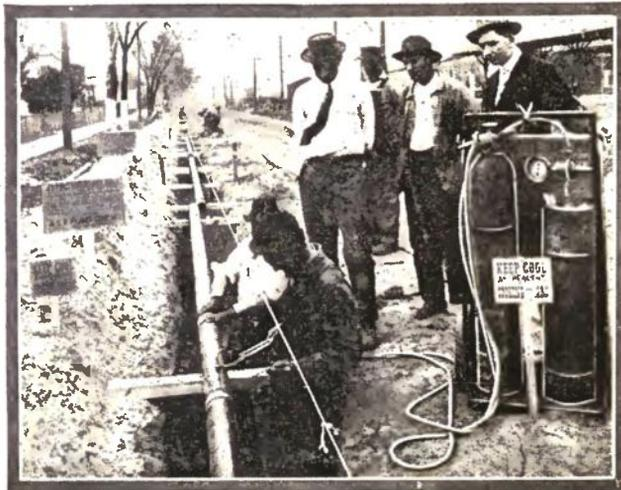
The Modern Way of Laying Gas Pipe is to Weld the Separate Lengths Together So as to Form One Continuous Piece of Metal.
