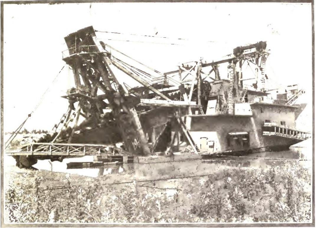
Claimed to be the Largest and Most Powerful in the World, this Dredge is Being Used in California for the Recovery of Gold. The Dredge has 87 Buckets of 16 Cubic Feet Capacity Each and is Electrically Operated.
