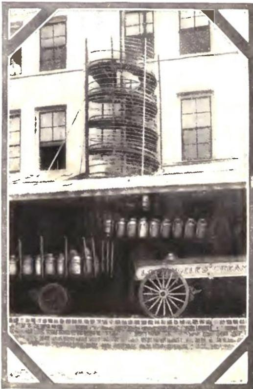
Much Time in the Handling of Milk Cans is Effected with the Use of a Spiral Can Slide.
