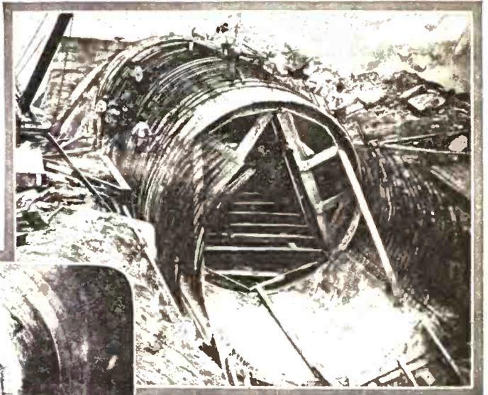
Above: Forms and Reinforcement Rods in Place, Prior to Pouring the Concrete for One of the Meter Tubes. At the Left: Looking Through the Throat Section of the Largest Water Meter in the World.
