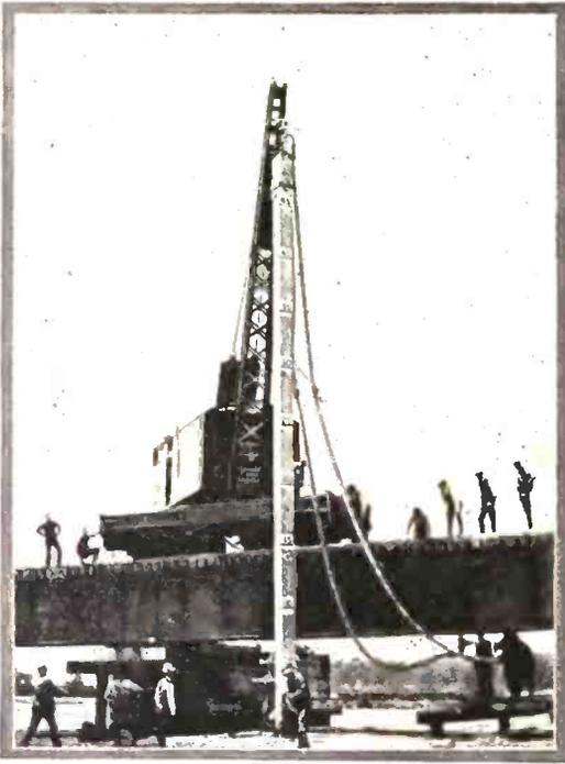
The Many Difficulties of Pile-Driving Have Been Eliminated in This New Pile Which Bores Its Own Hole.
