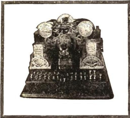
Front View of the Automatic Receiving Set: The Main Motor may be seen in the Center, and the Variable Condensers on Either Side of It. The Key-board is Placed in Front.
