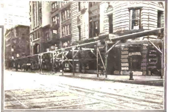
Two Views of the Wooden Trestles Which Carry the Gas Pipes Over the Streets During the Construction of New York's Subways. These Overhead Pipes Have Eliminated the Danger of Explosions Due to Leaking Pipes.
