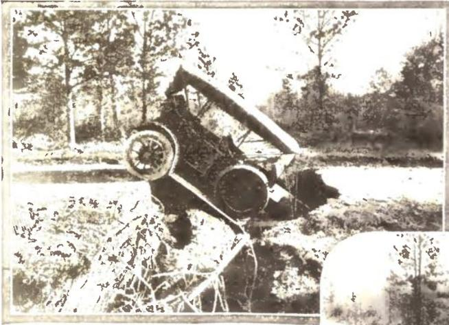
Two Views of a Strange Accident that Befell a Powerful Touring Car. Although the Automobile Made a Large Hole in the Ground, the Only Damage it Sustained was in the Form of a Bent Front Axle and Damaged Front Mud Guards.
